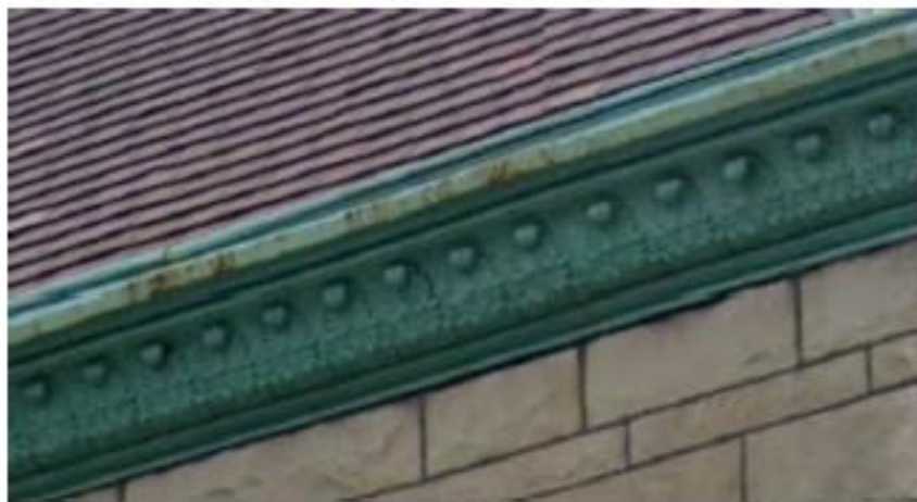
FIX / BEND / PATCH CORNICES, THEN PAINT PATCHES TO EITHER MATCH EXISTING GREEN COLOR OF COPPER OR MATCH EXISTING BROWN COLOR OF COPPER DOWNSPOUT
