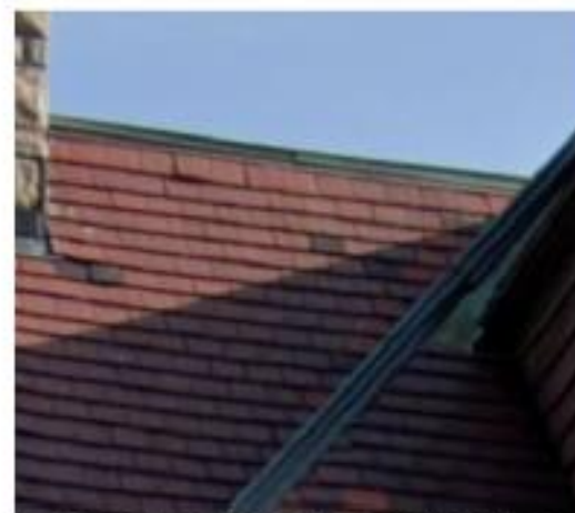
REPLACE NECESSARY ROOF TILES AND COPPER WORK FOR ROOF TO MATCH EXISTING
