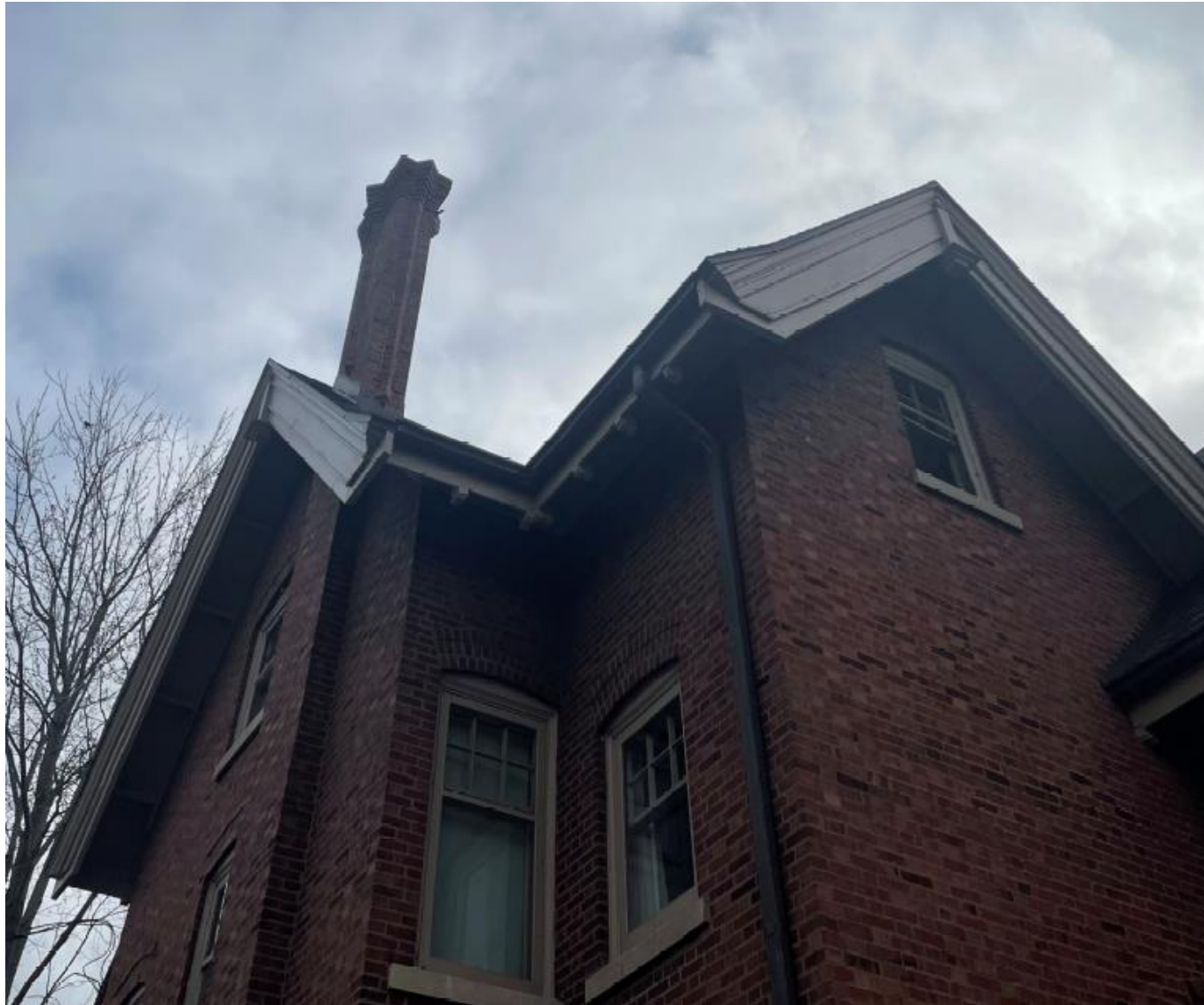
The main chimney will be re-built to match the top of the west chimney
