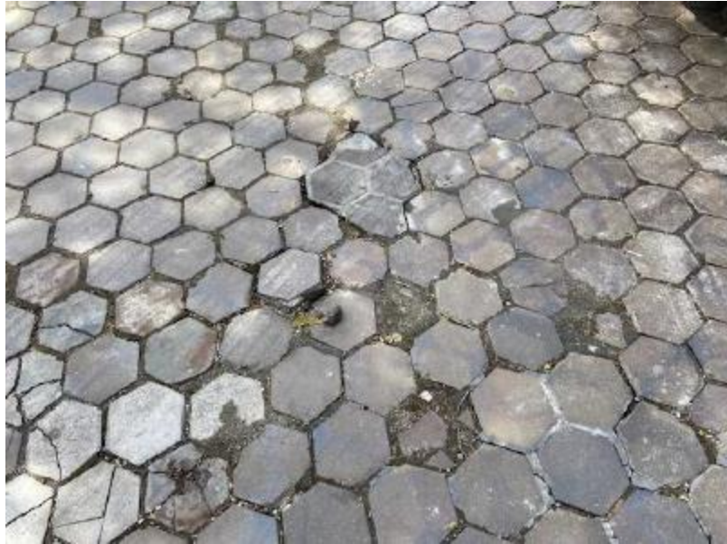
Examples of driveway tile deterioration
