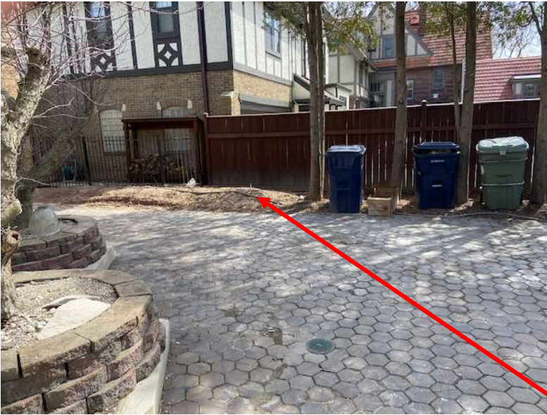
Dirt area where pad will be poured for storage of carts. Note that currently they are on mud between the trees. Pad will be hidden by portico so carts will be concealed from the street.
