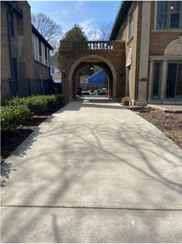
Existing Concrete Driveway: Facing West from Front of house
