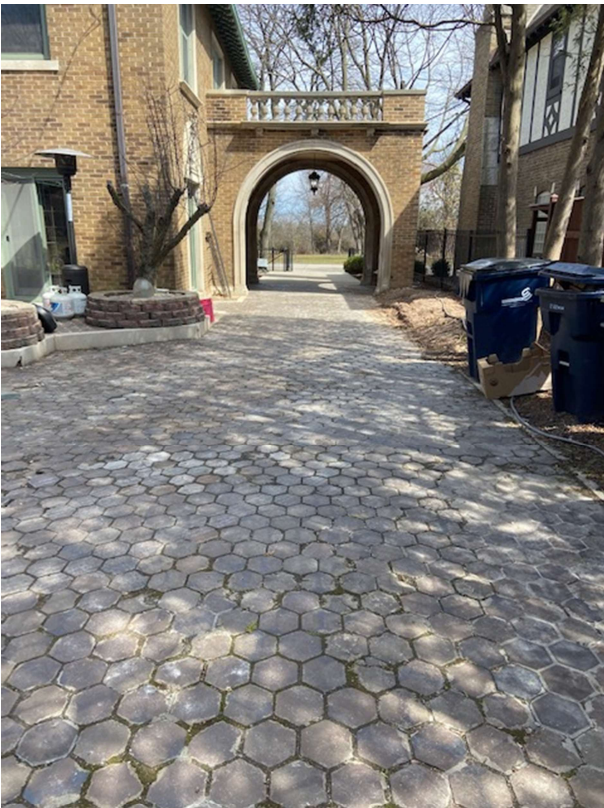
Rear Driveway: Existing Tile - Facing East
