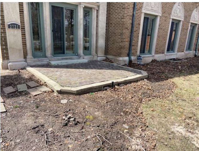
Front Patio showing deterioration – Note paving stones connecting patio to driveway.
