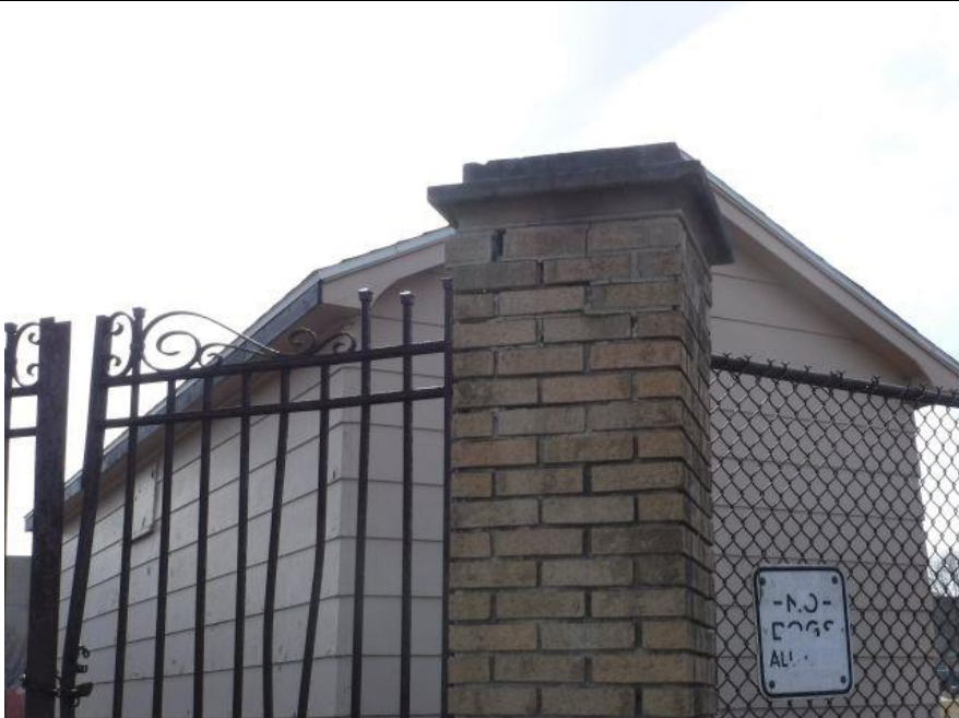
Photo 71 Northeast iron gate to be painted and top of columns repaired
