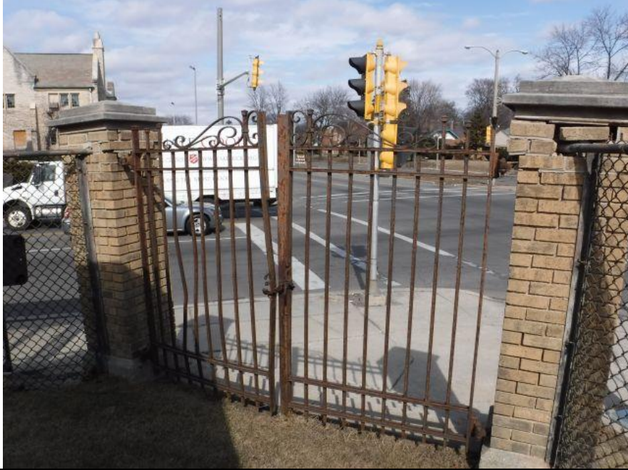
Photo #31 Iron Gate at NE corner – gate to be painted – top of columns repaired
