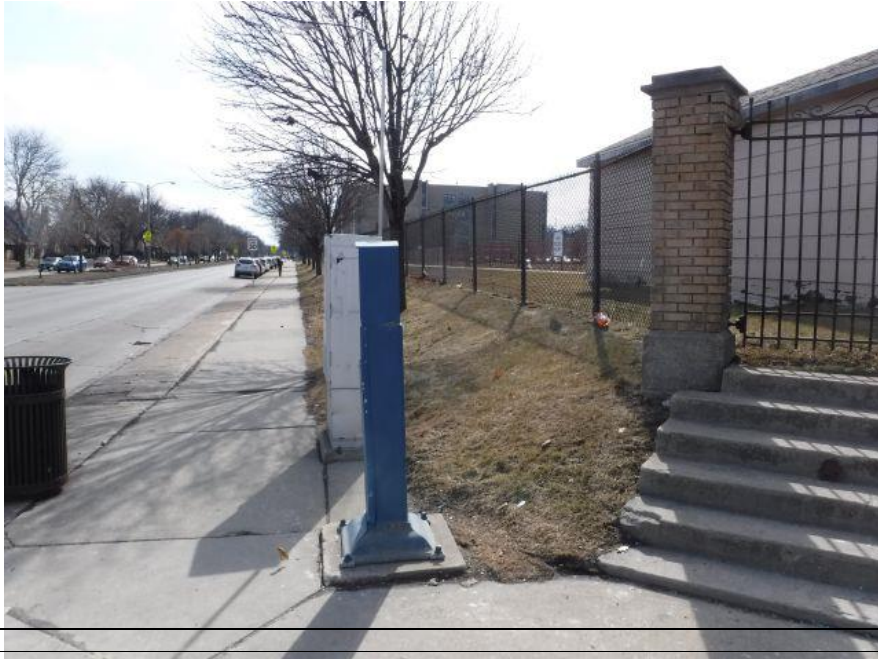
Photo 71 Northeast iron gate to be painted and top of columns repaired
