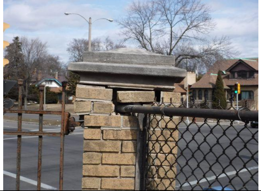
Photo #32 Iron Gate at NE corner – gate to be painted – top of columns repaired
