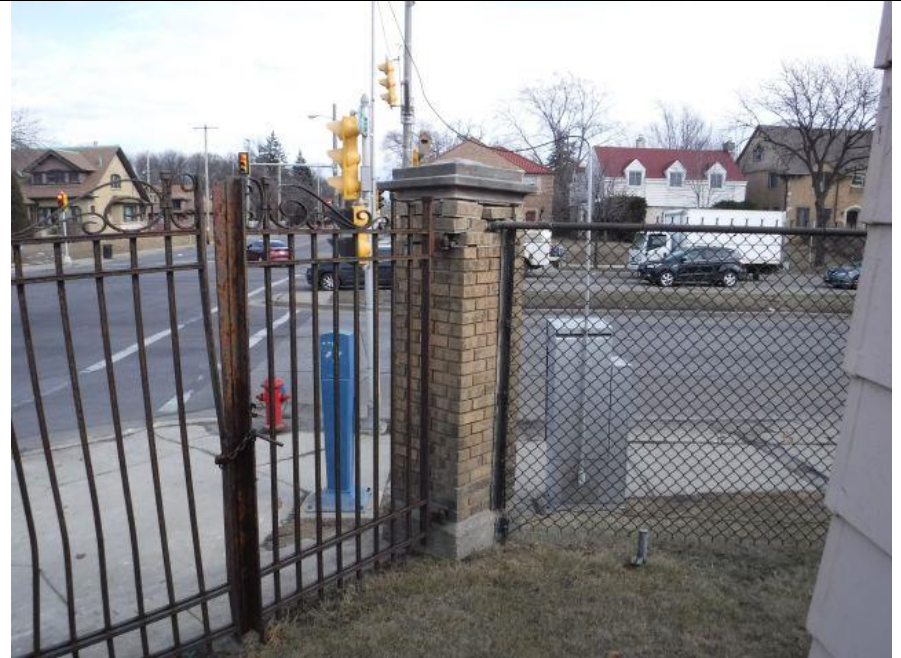
Photo #36 Iron Gate at NE corner – gate to be painted – top of columns repaired
