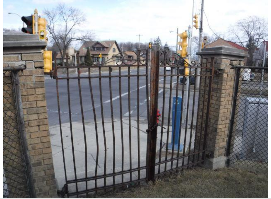
Photo #36 Iron Gate at NE corner – gate to be painted – top of columns repaired
