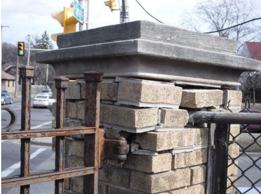
Photo #31 Iron Gate at NE corner – gate to be painted – top of columns repaired
