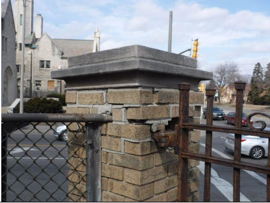
Photo #35 Iron Gate at NE corner – gate to be painted – top of columns repaired
