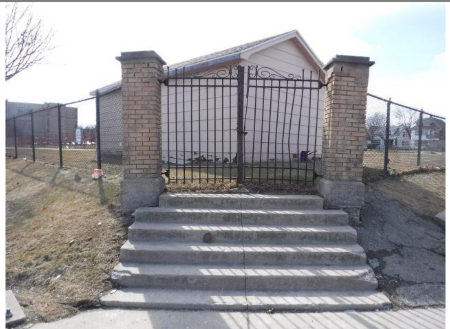
Photo #68 Northeast iron gate to be painted and top of columns repaired
