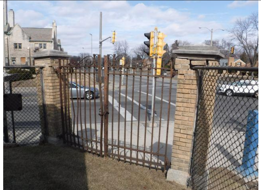
Photo #28 Iron Gate at NE corner – gate to be painted – top of columns repaired
