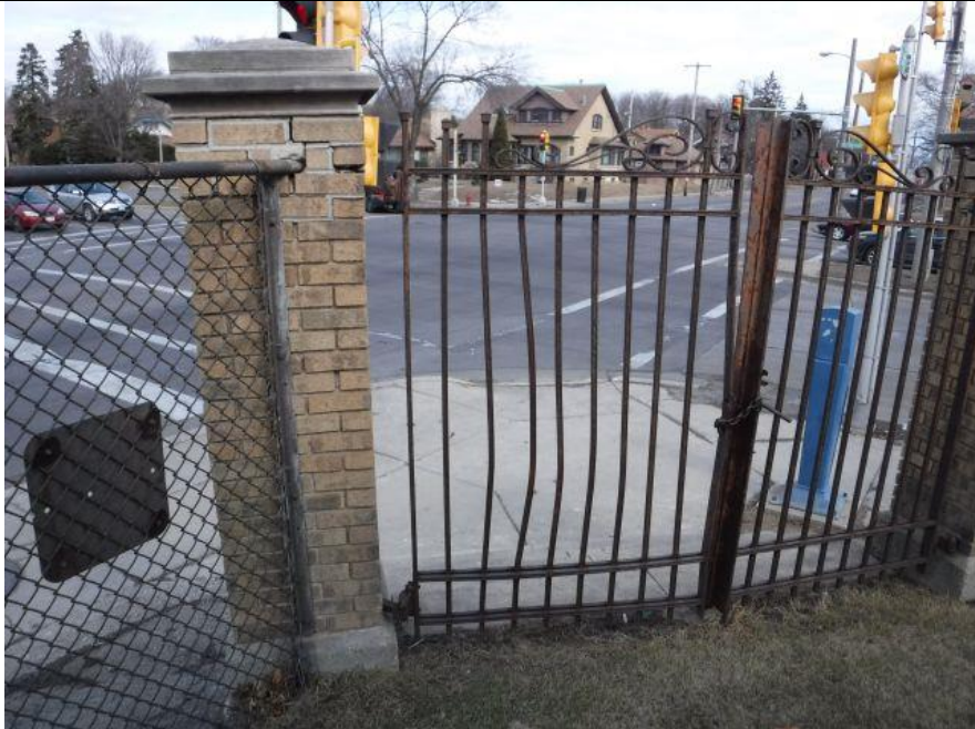
Photo #35 Iron Gate at NE corner – gate to be painted – top of columns repaired
