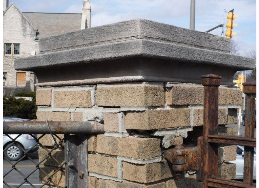
Photo #32 Iron Gate at NE corner – gate to be painted – top of columns repaired
