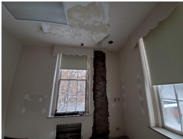
Photo 19: Deteriorated wall and ceiling in Northwest Quadrant.
