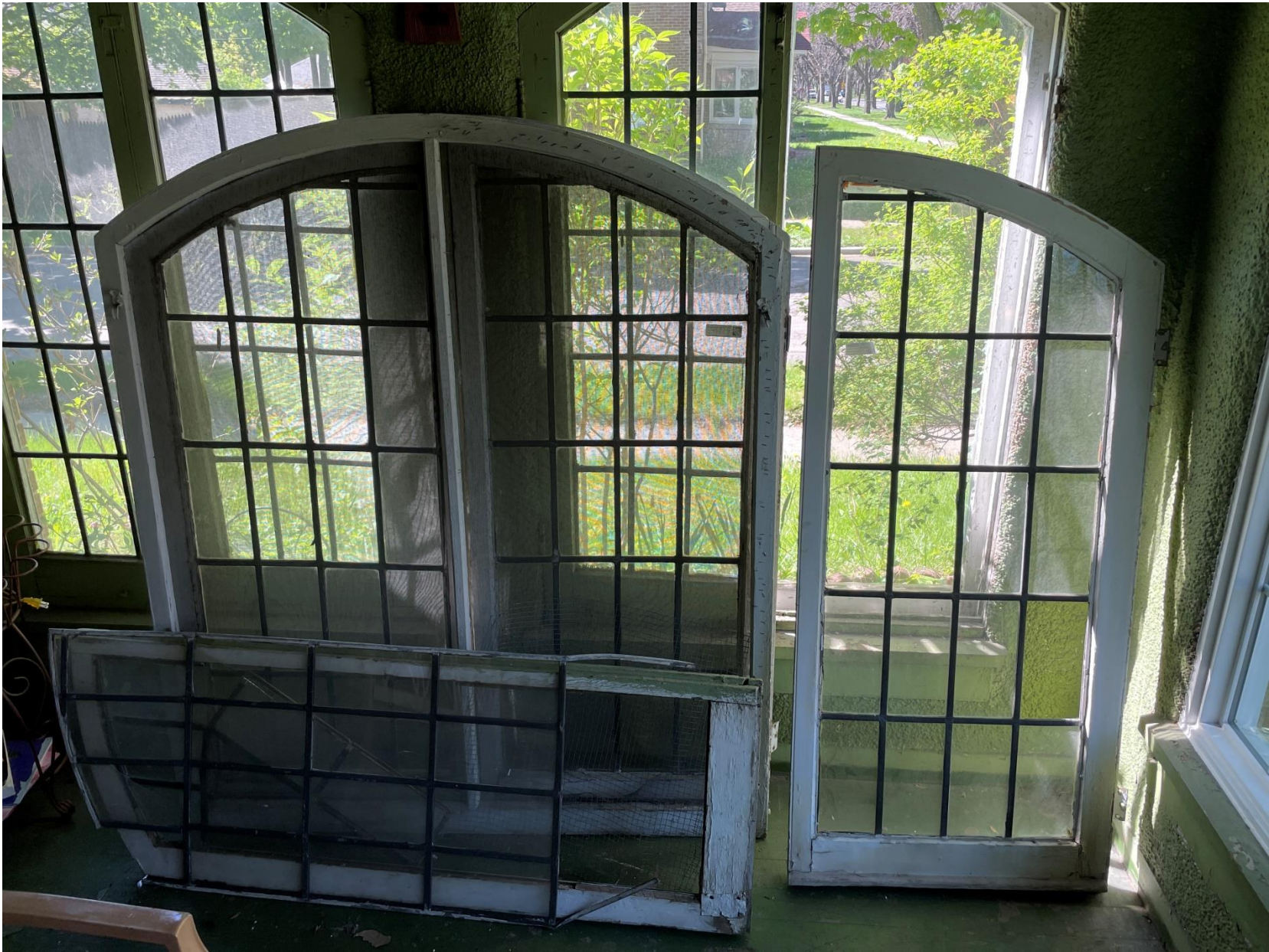
Photo of original windows to be restored and re-installed.
