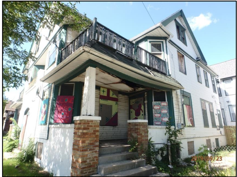
Photo of multi-unit building to be demolished (2019)
