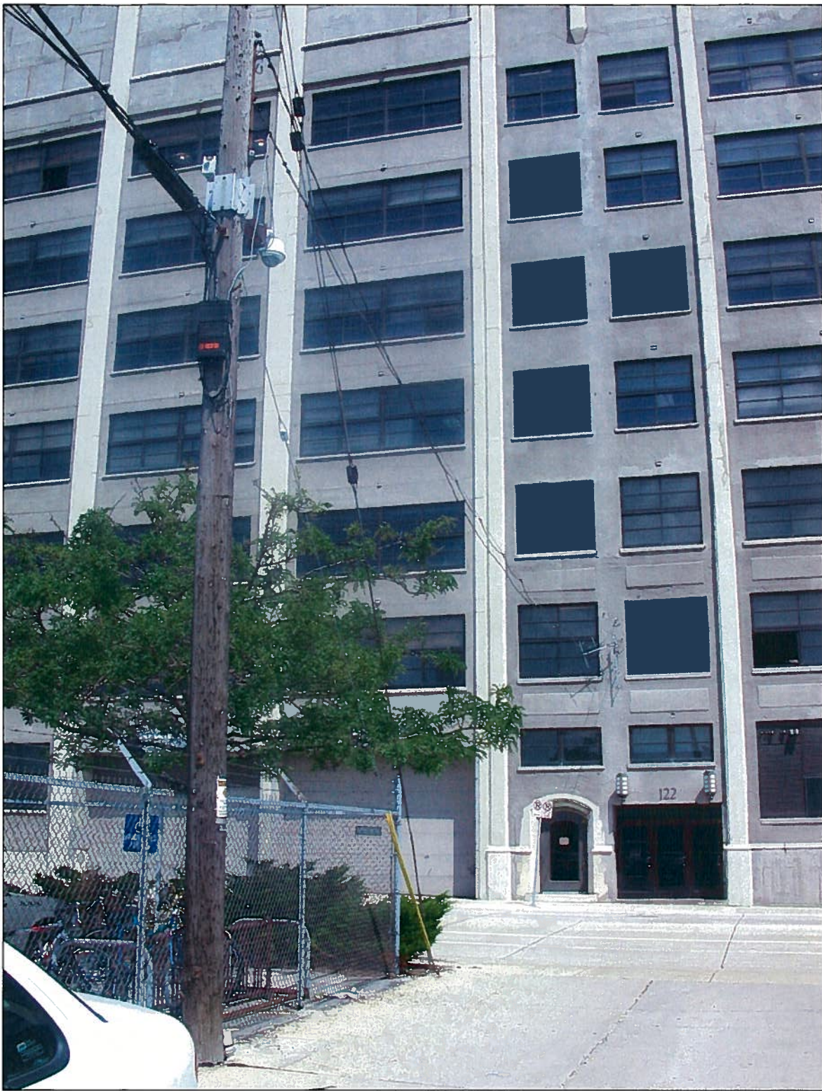
CCF 091125 136 W Greenfield Ave 7-23-10 Looking N towards Greenfield Ave at security camera and overhead cables for camera.
