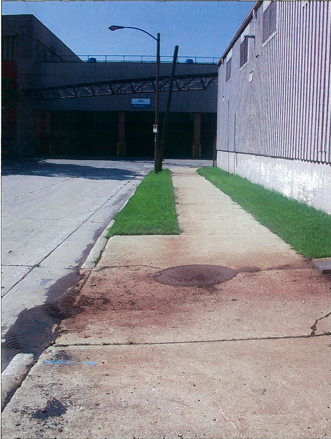
CCF 091125 136 W Greenfield Ave 7-23-10 Looking S towards vacated Lapham St at manhole in W sidewalk of S Barclay St.
