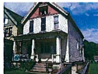
65 100_3156 6/22/2009 Taken By: Chad Frost 2222 Rec Center
