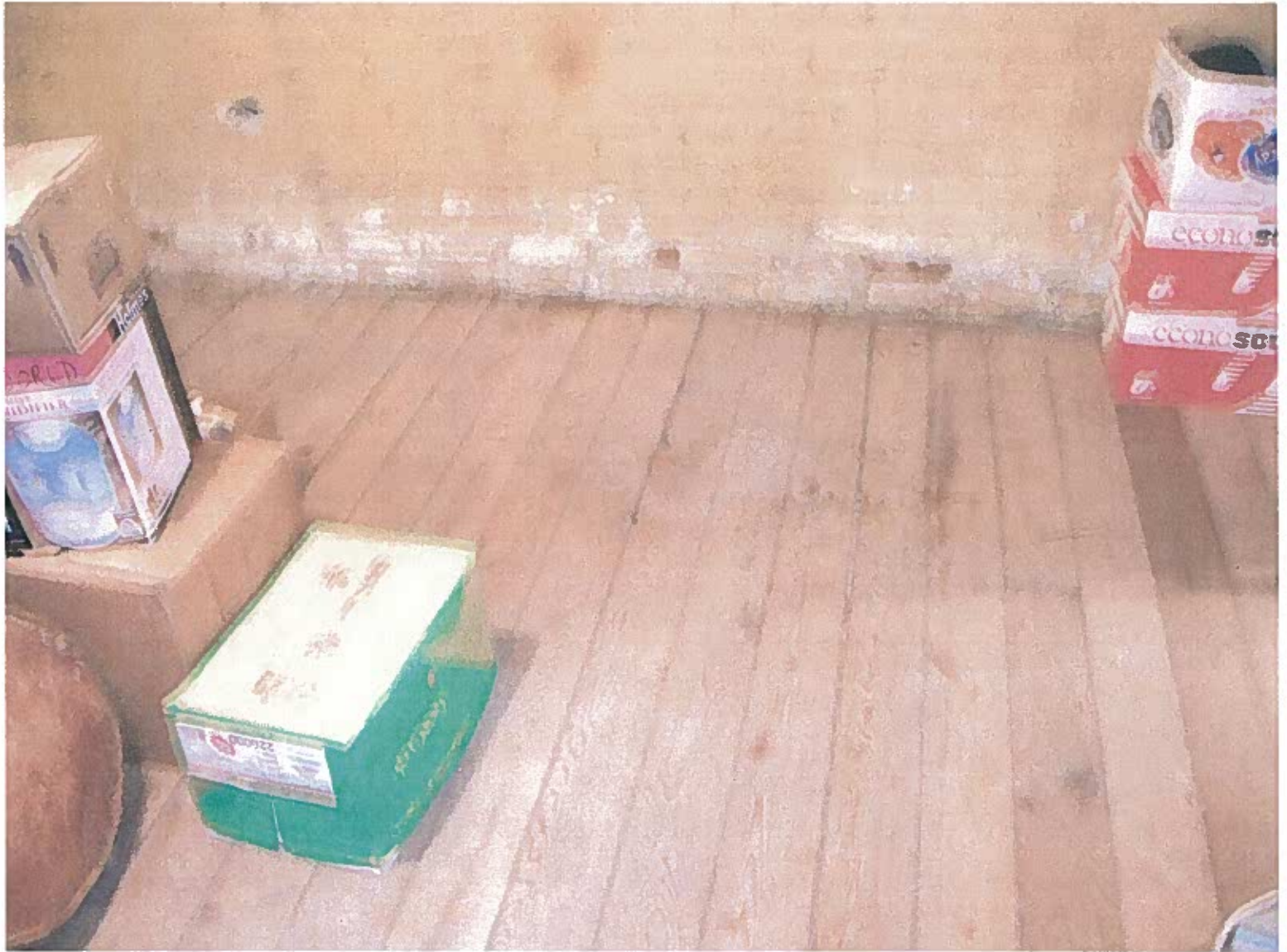
Storage room Floor and raw earth under, were Staturated with Sewage.
