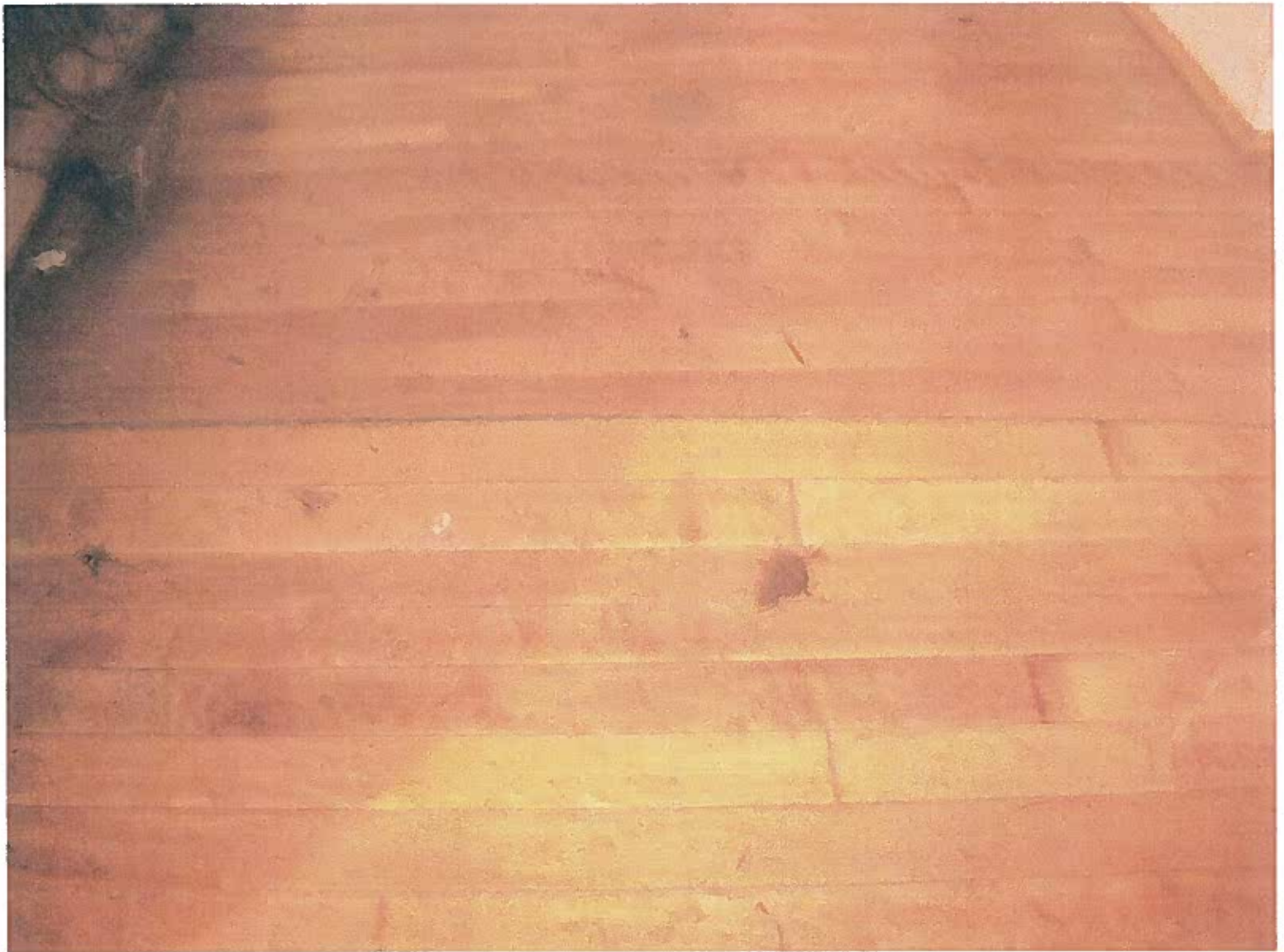
Floor completely warped and buckled.
