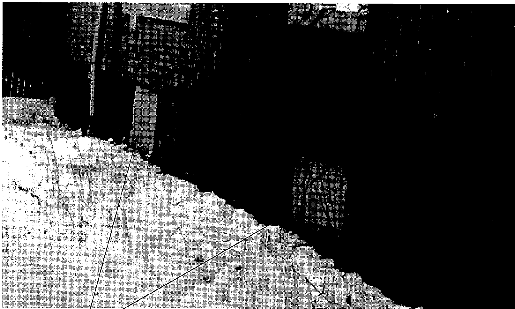
Boarded-up basement windows around the house to be opened up and fitted with new wood jambs, sash and storm
