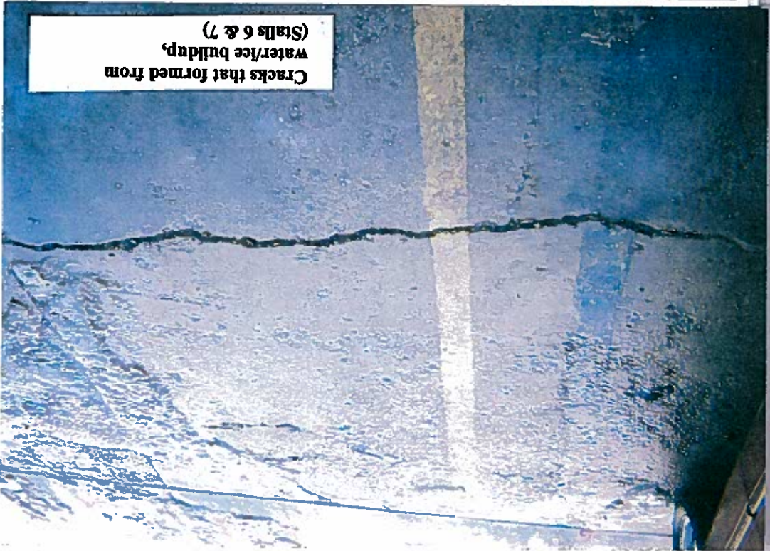
Crack caused by settled ice, (Stall 8)
