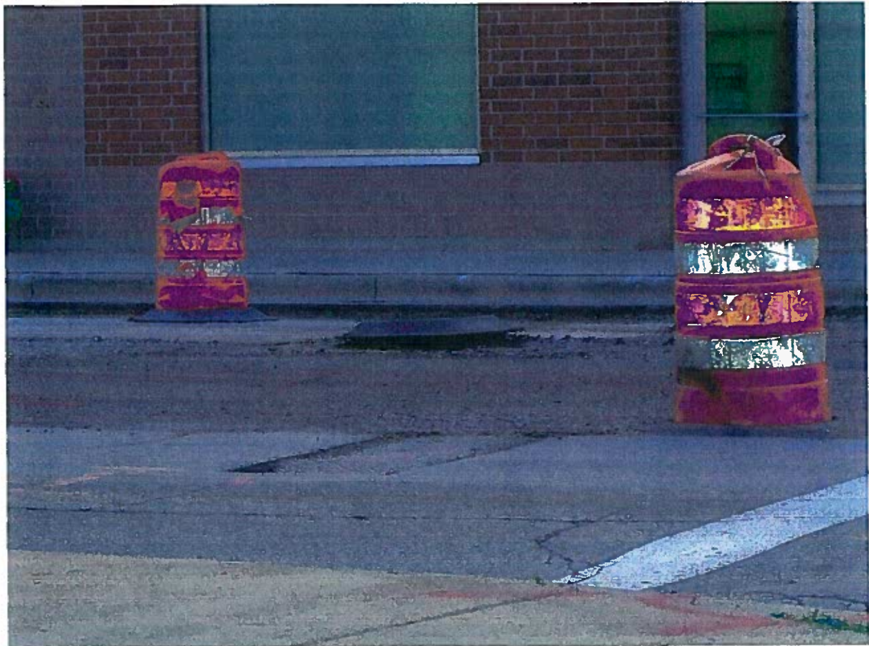
Attachment A: A protruding manhole cover marked only by a black ring.
