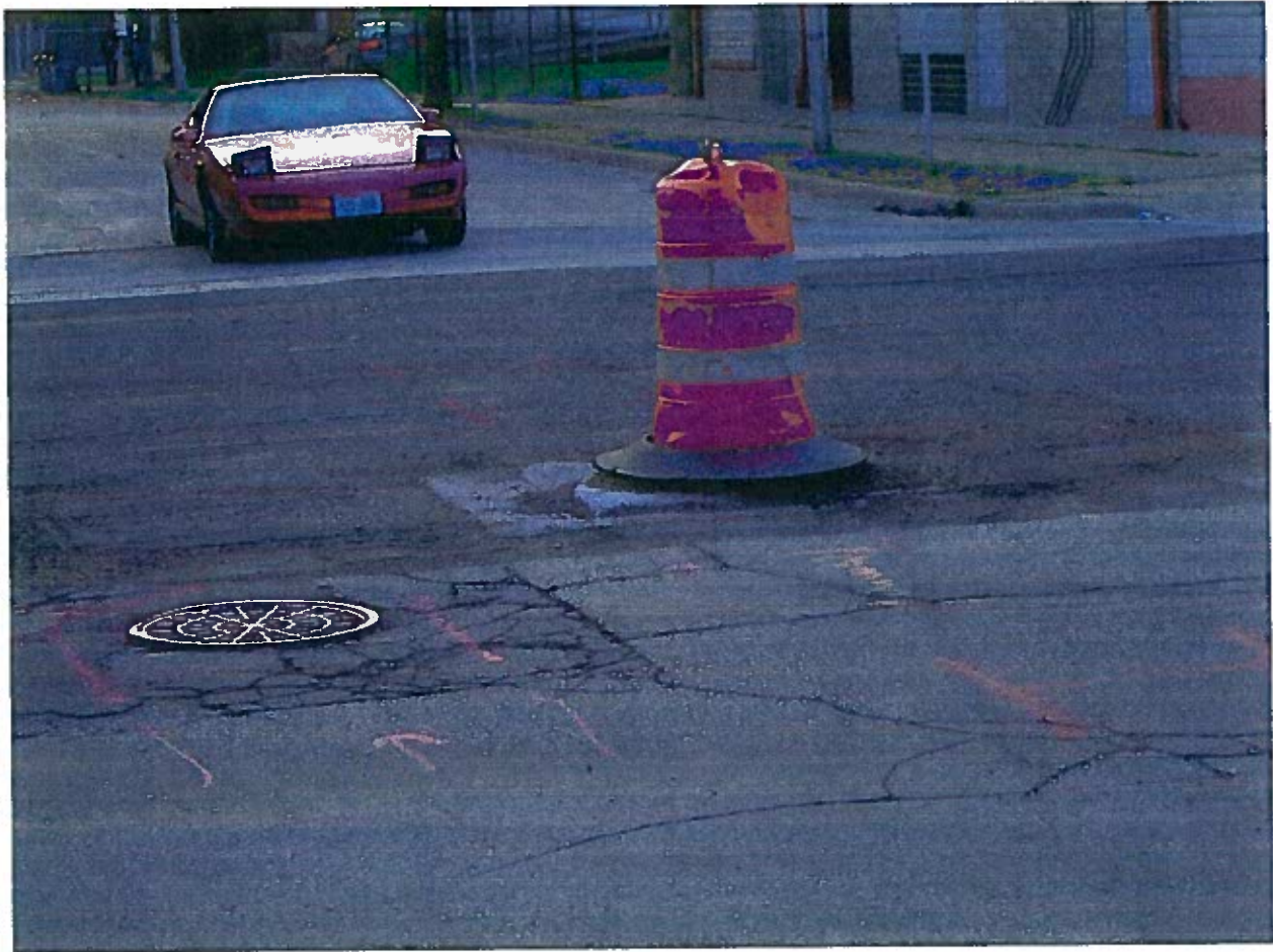
Attachment B: A dented orange barrel sits atop a protruding manhole cover as a vehicle attempts to navigate the intersection.
