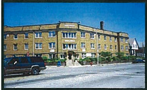
UMCS Existing Facility
