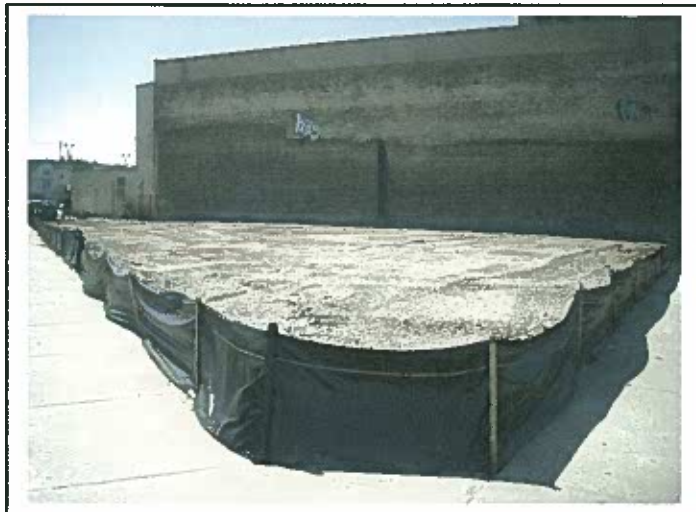
Pic #1 - Looking South West
