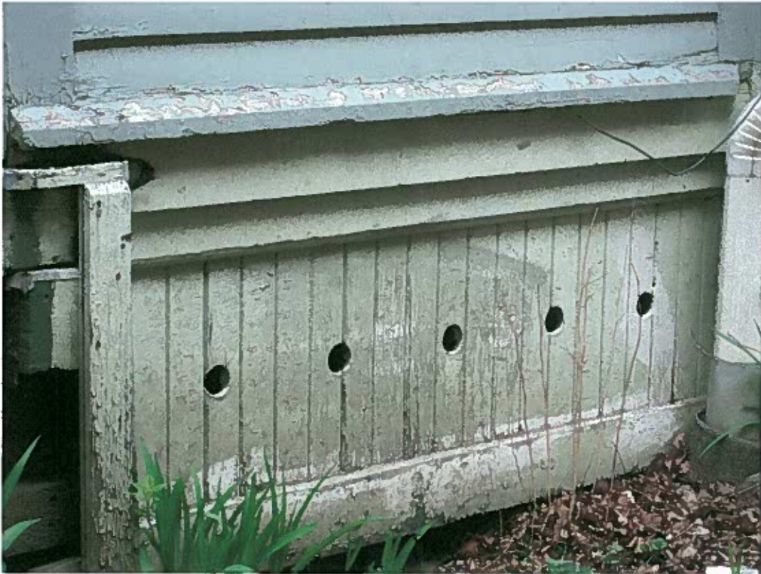
5. Solid Board skirt below Front Entry foyer
