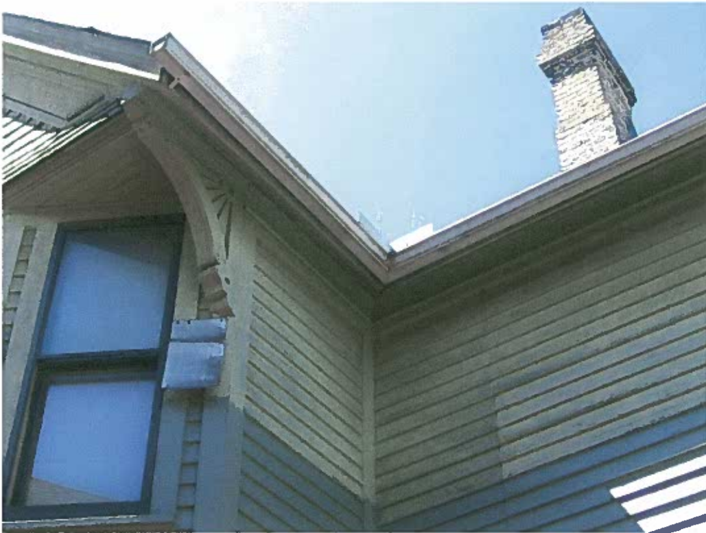
7. Second floor (North-East Elevation) above side porch
