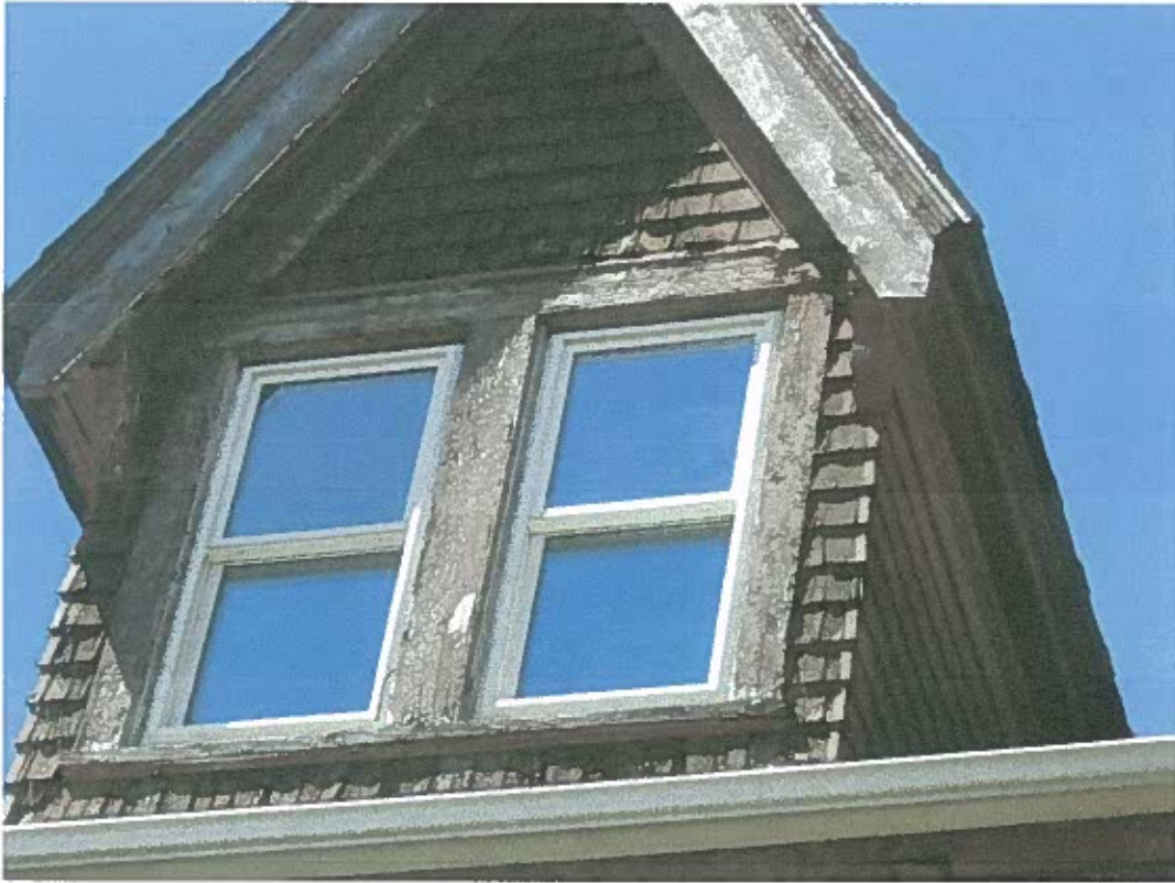
6. Northern-most Attic Dormer with wood shingle details above new K-Style gutter
