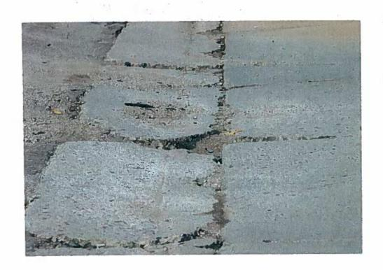
This picture is a closer view of the shoulder and the pothole. As can be seen by this picture, the entire shoulder of the street is dilapidated.
