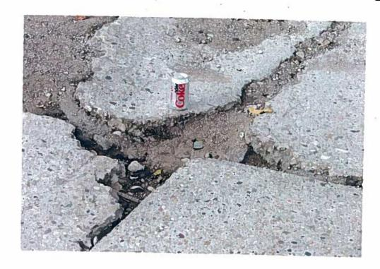
5) This is a much closer picture of the pothole. One can get an idea of the size of it by comparing the diet coke can to it. The depth of the pothole ist about 5-51/2 inches.
