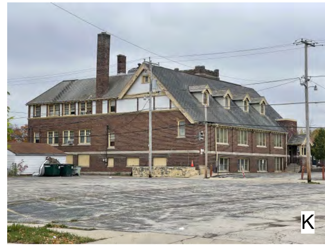
ALLEY VIEW: REAR OF ST. MATTHEW CME CHURCH, 2944 N. 9TH ST
