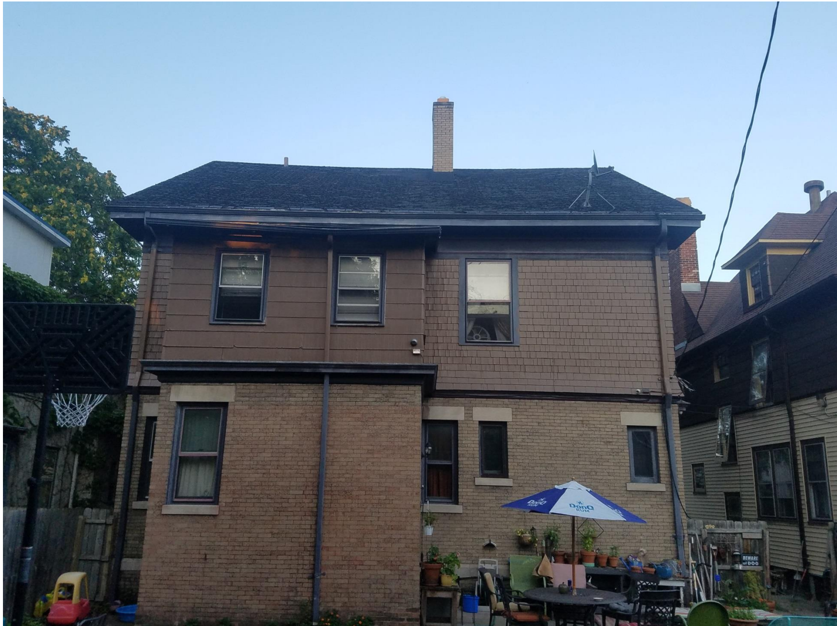
Current back view of house.
