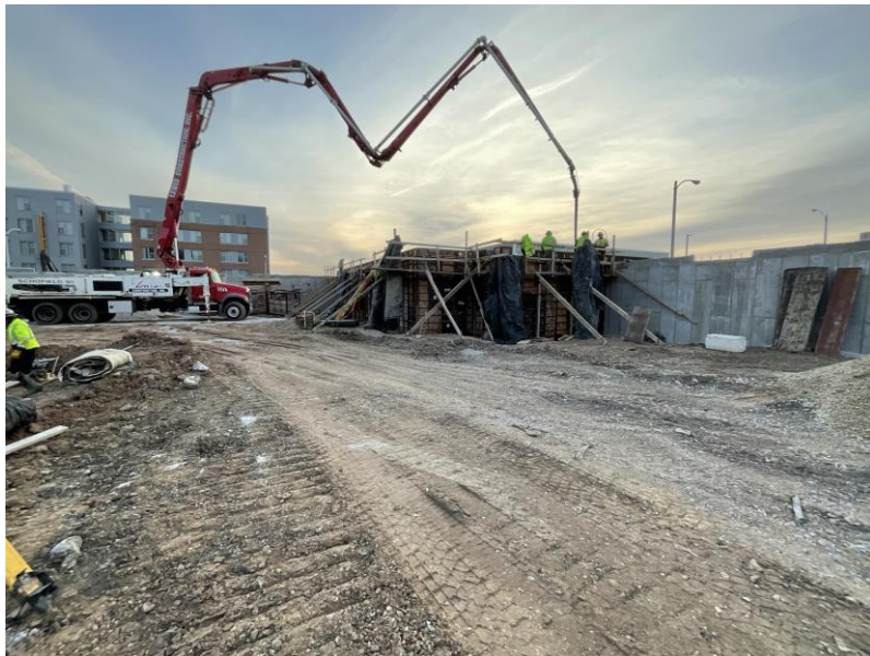
Pumping of concrete for building foundation
