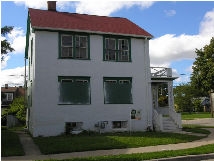
After exterior rehabilitation.
