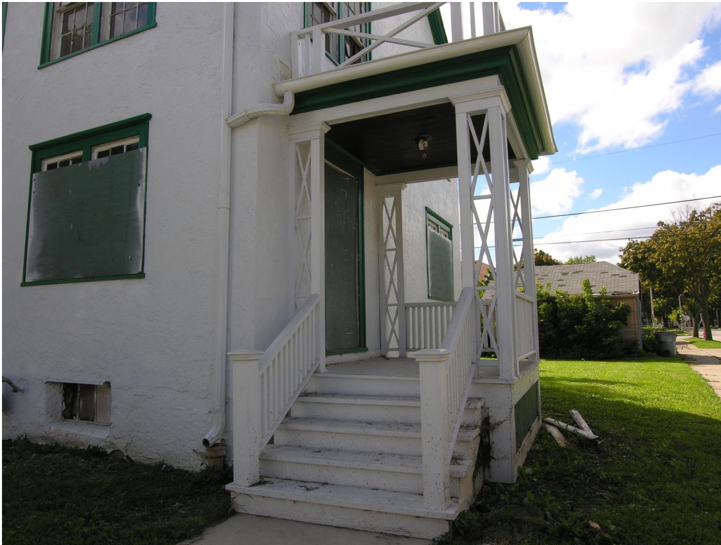
After exterior rehabilitation.
