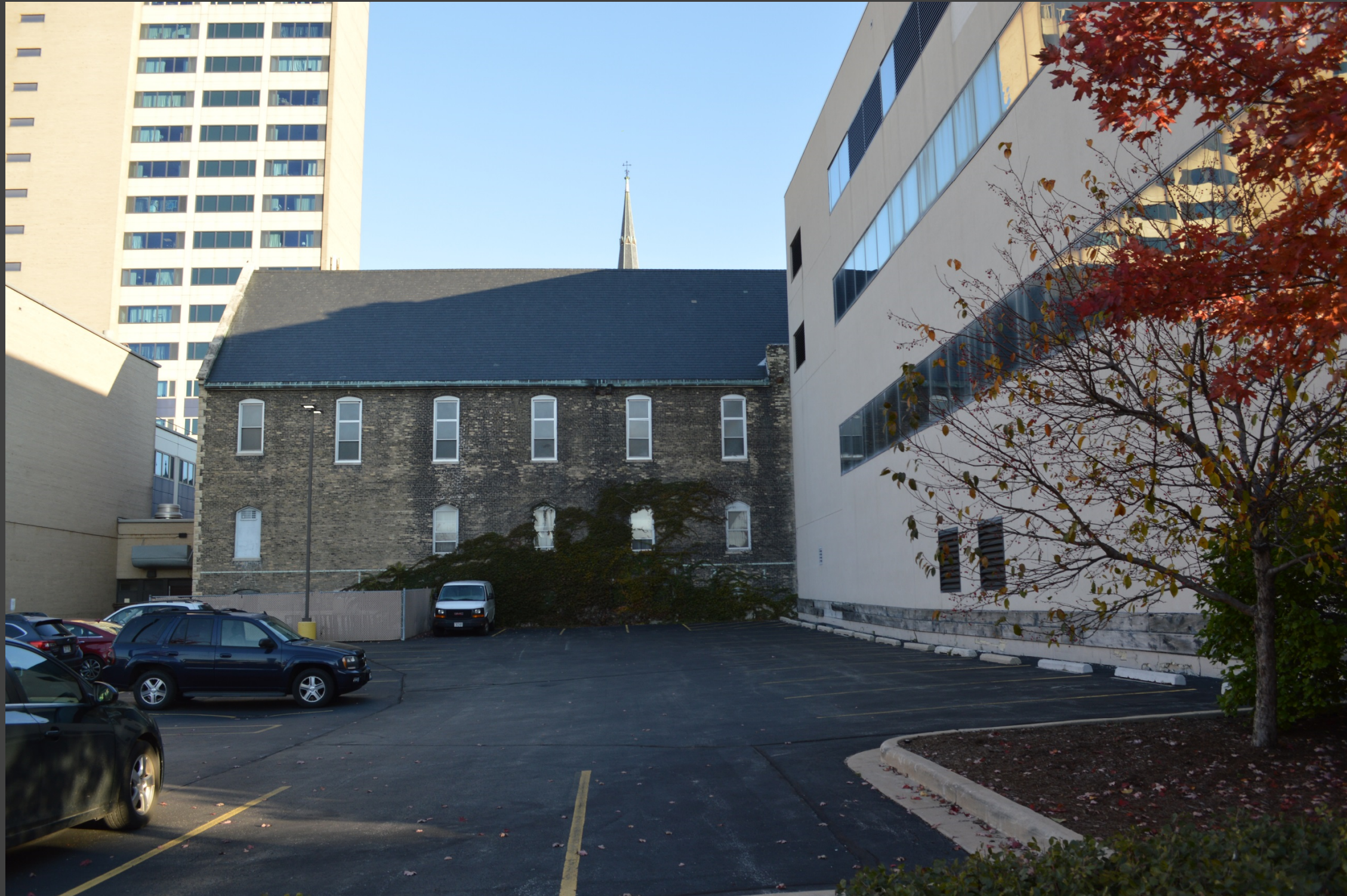
PARISH HOUSE SOUTH FACADE
