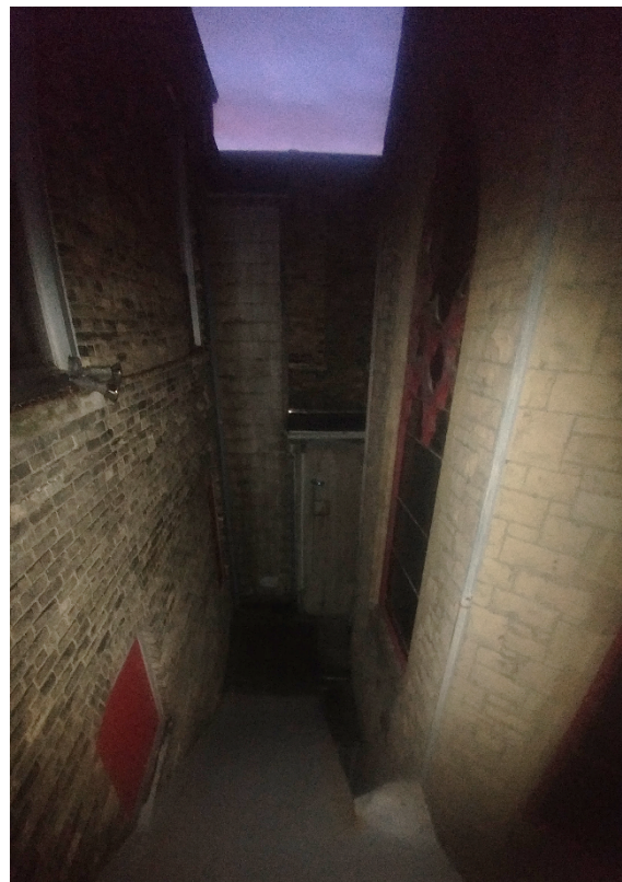
EXPOSING THE APSE INSIDE THE ADDITION
