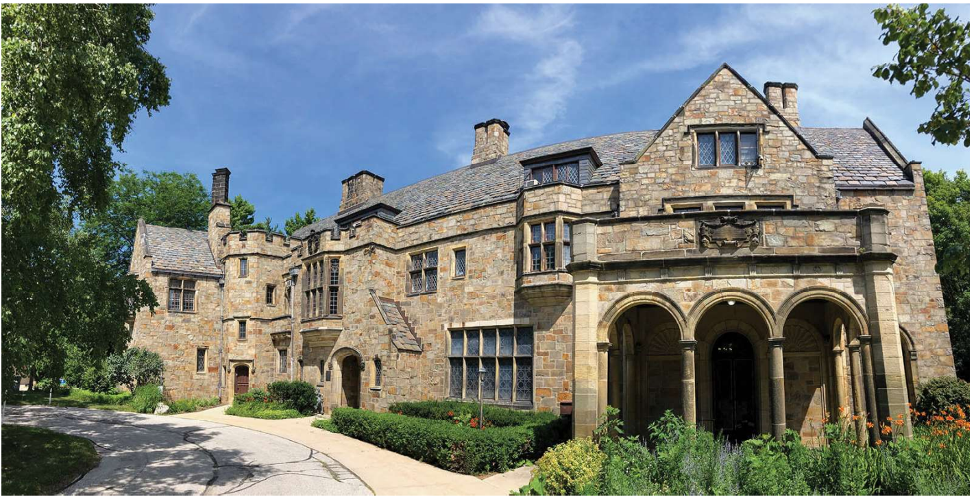
3. Exterior West View
