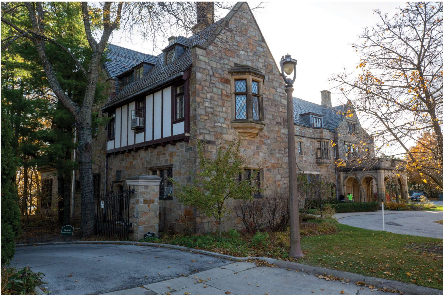
5. Exterior View from NW
