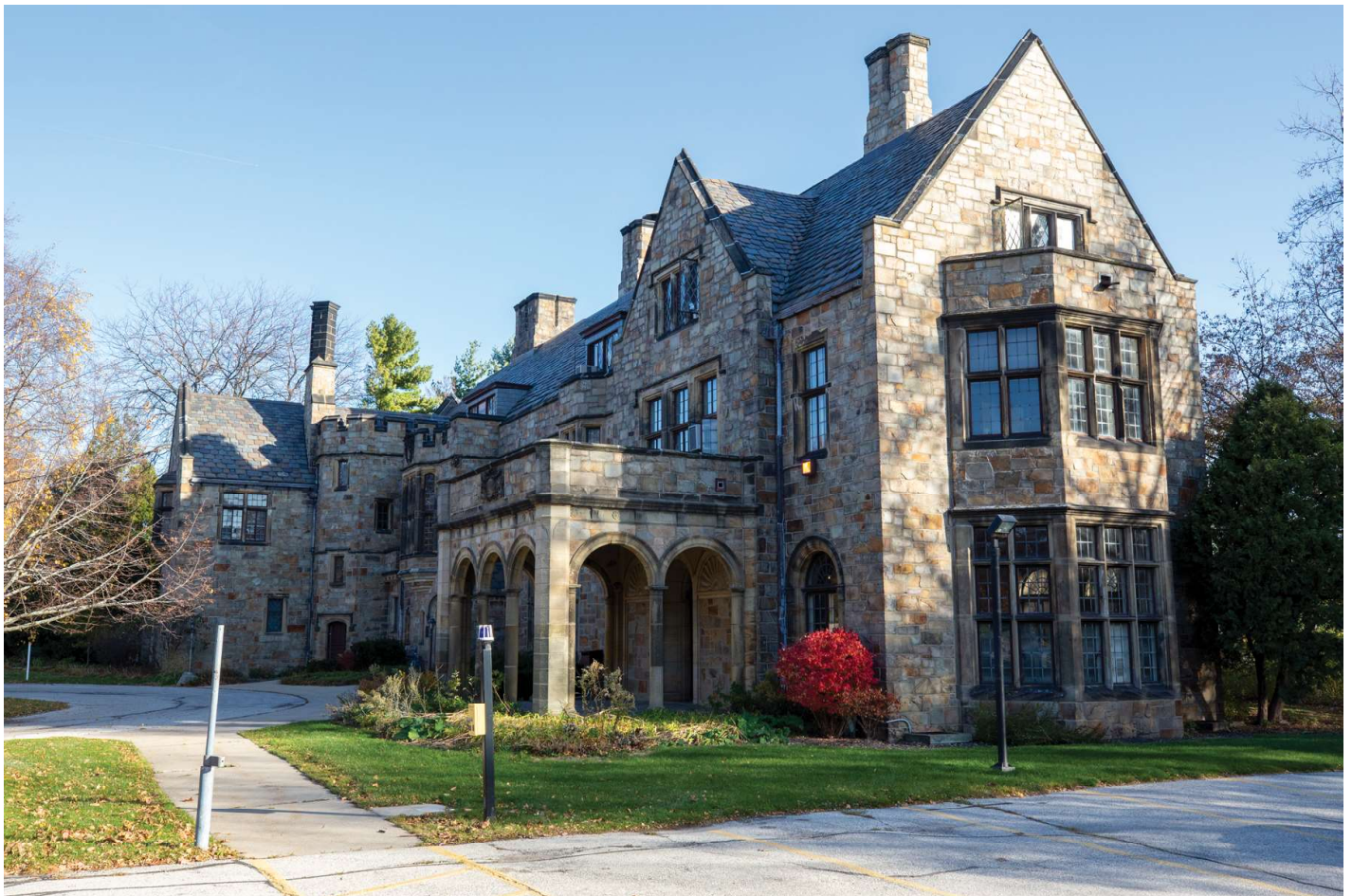
2. Exterior View from SW
