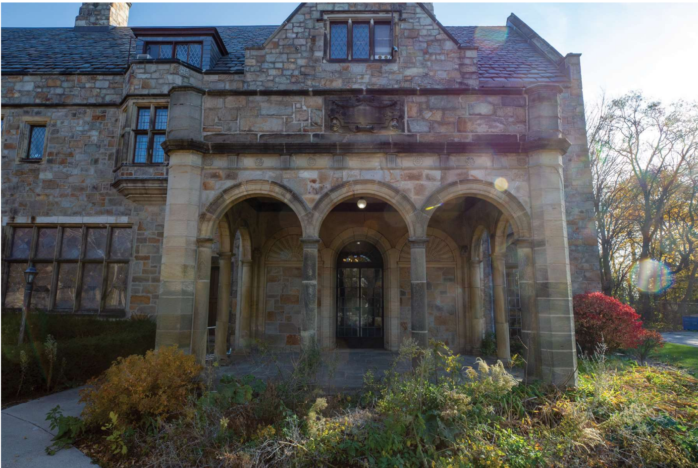
14. Porch off West Wall of Garden Room
