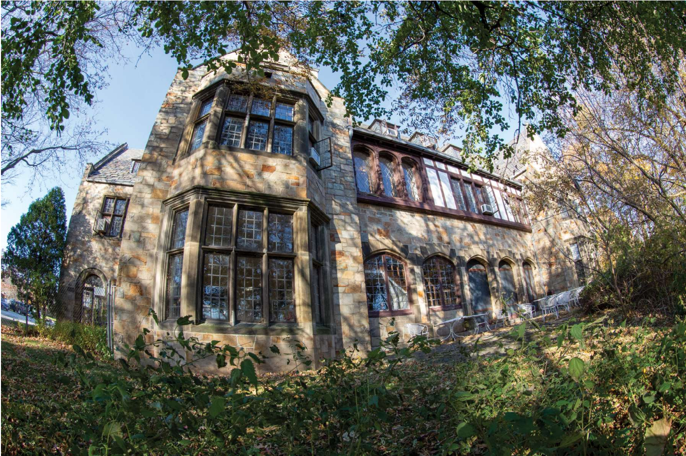
11. Exterior View from East Shading Toward SE Corner
