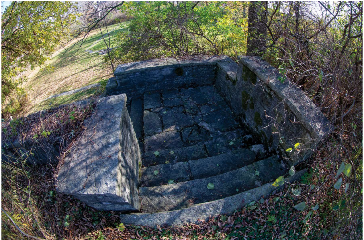
51. Stone Staircase from West to the Pool
