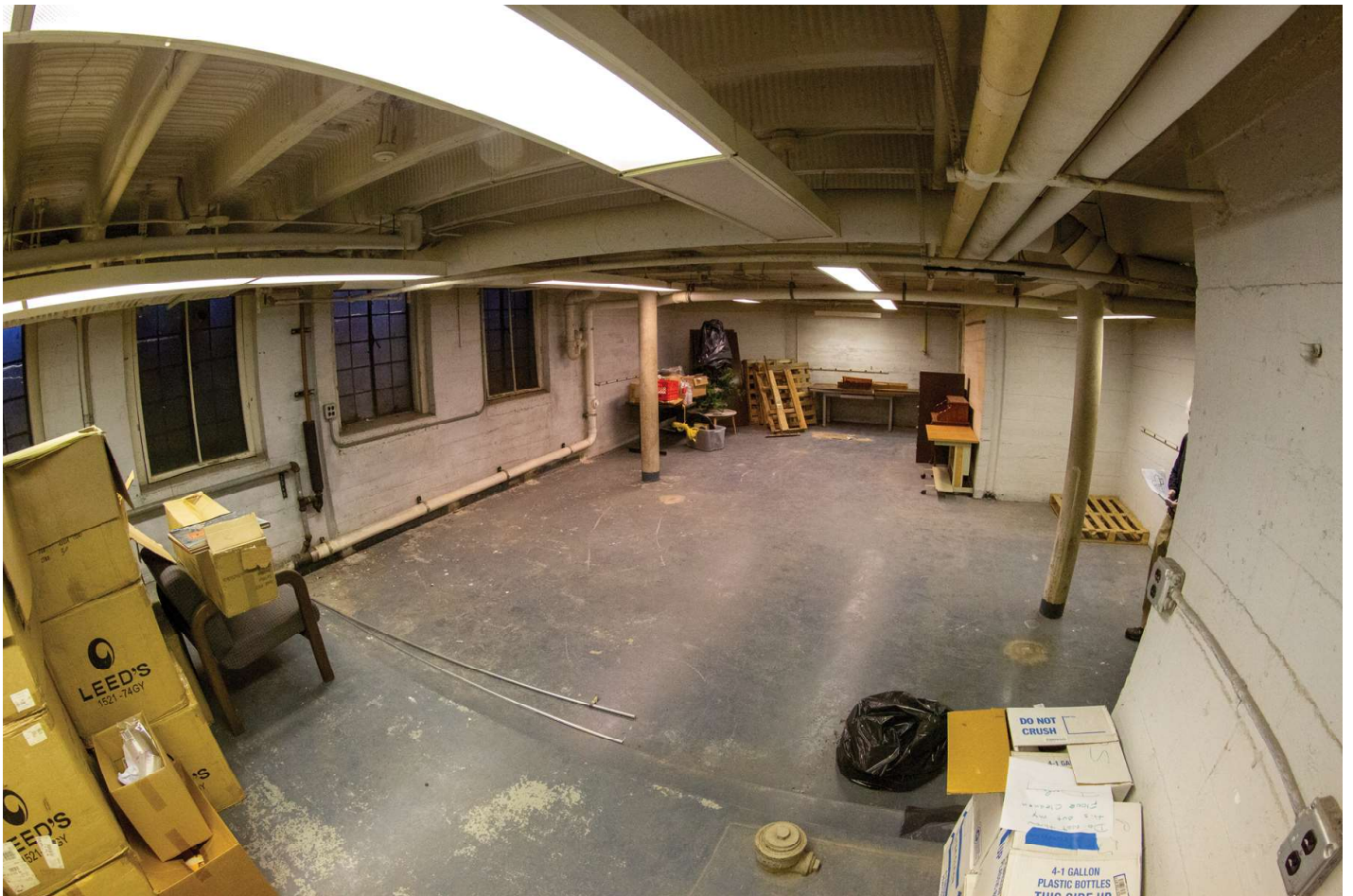
35. Laundry Room from SW Corner
