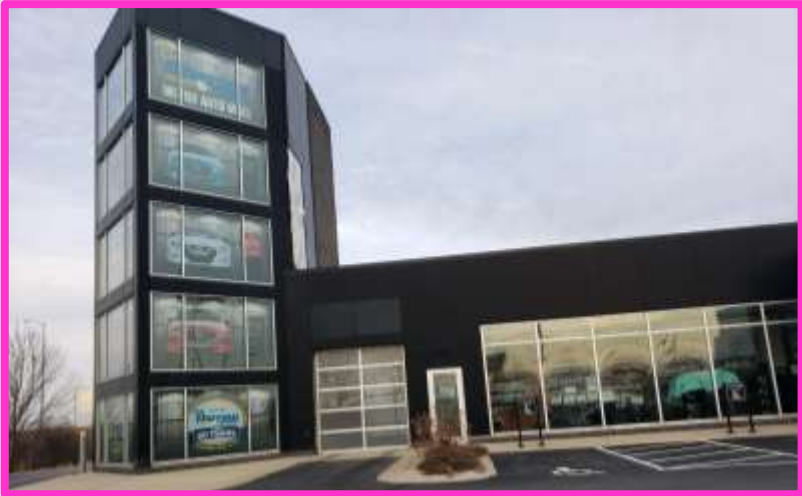
View of former Smart Car tower looking northeast
