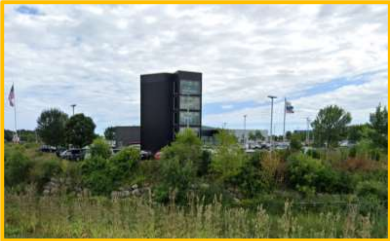
View from Good Hope Rd on-ramp looking southeast
