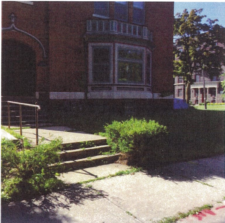
SHOWS THE BAY WINDOW WHICH THE NEW APPROACH WILL BE CENTERED ON
