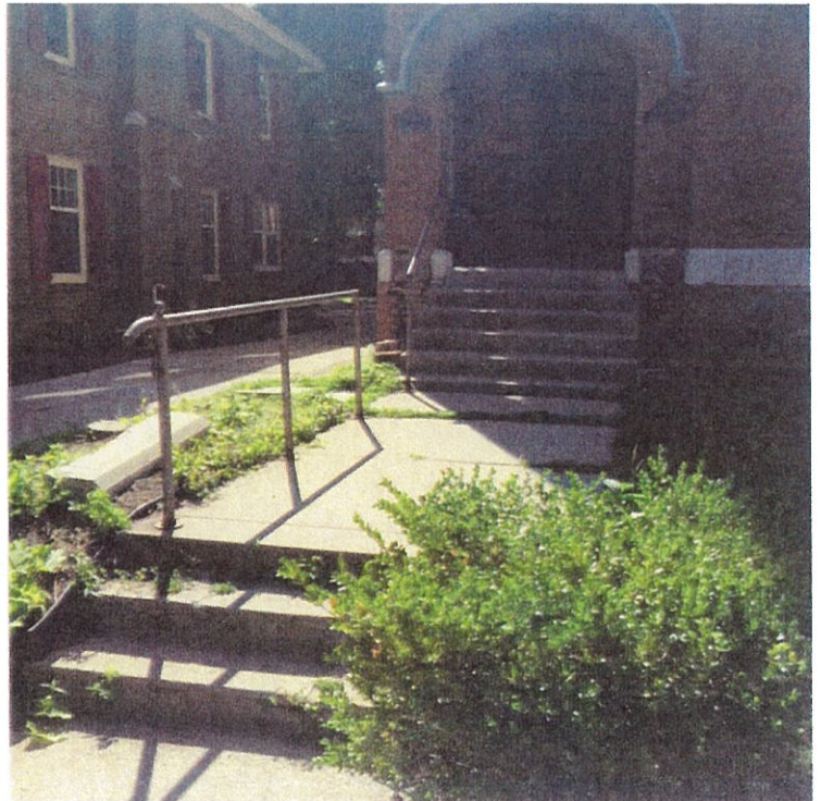
PHOTO OF EXISTING APPROACH + SIDEWALK
