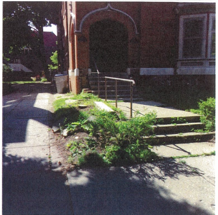
EXISTING SIDEWALK FROM HOUSE NOTE PROXIMITY TO NEIGHBORS DRIVEWAY
