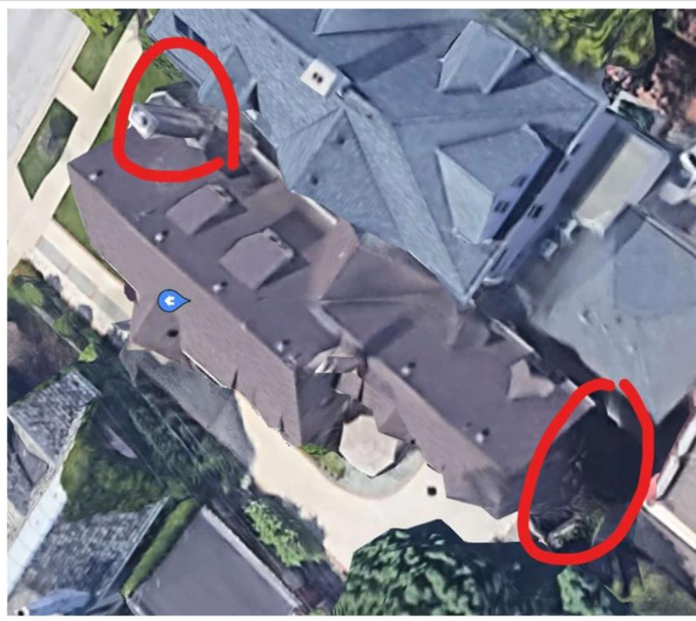
Figure 1. Overhead from Google Maps showing proposed location of compressor on the north facade and location of the chimney to be tucked-pointed.
