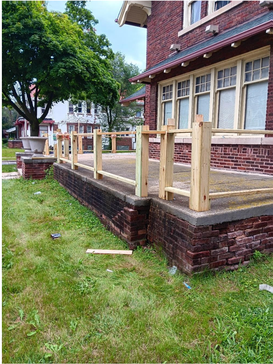
Existing porch condition
