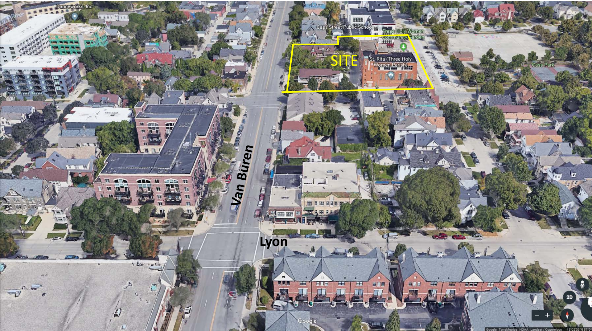
View looking North
