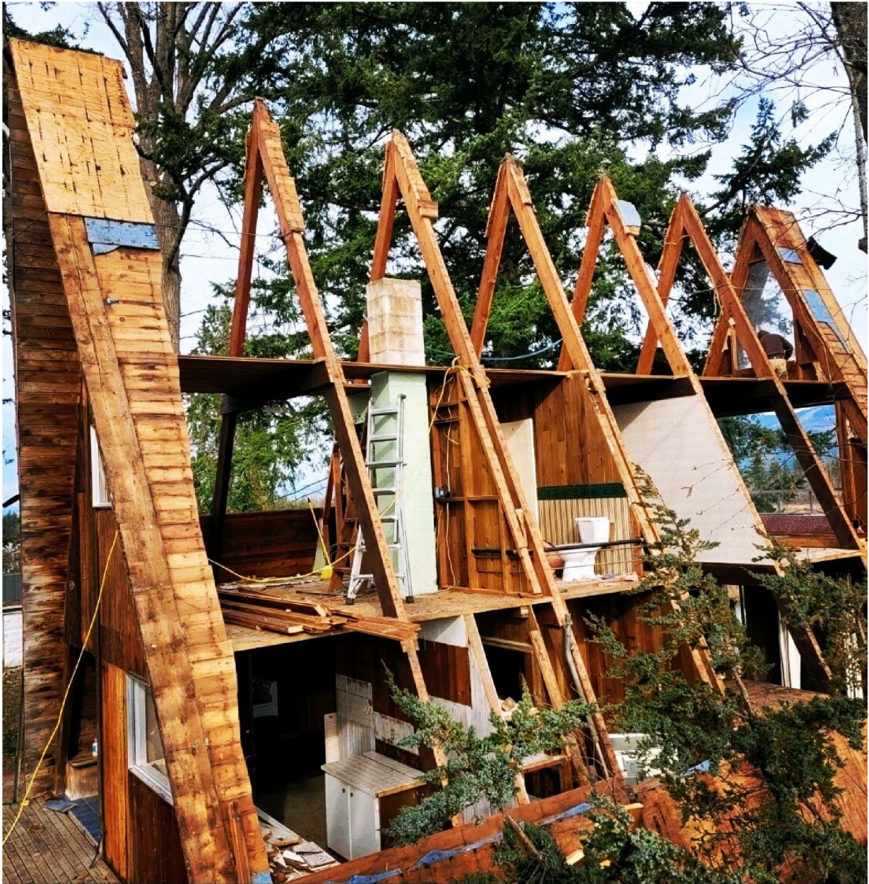
An A-frame home, mid-deconstruction. Photo courtesy Dave Bennink
