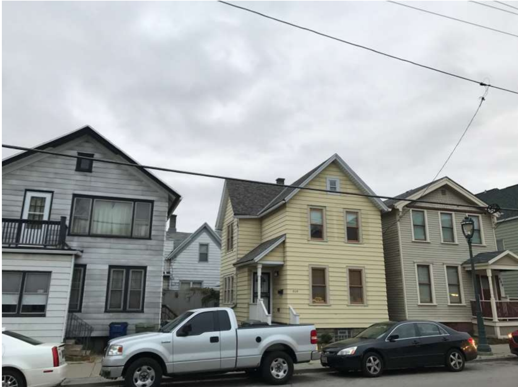
Overview at completion.
