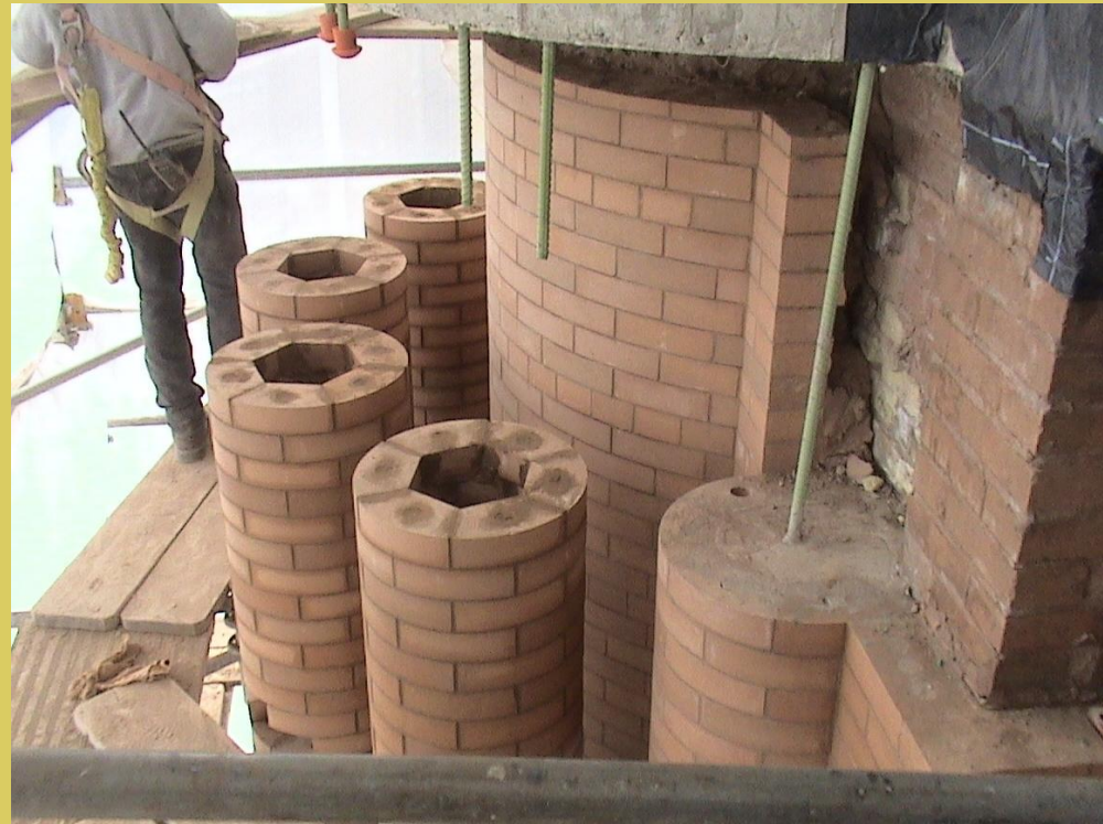
Continued brick work on the south tower.
