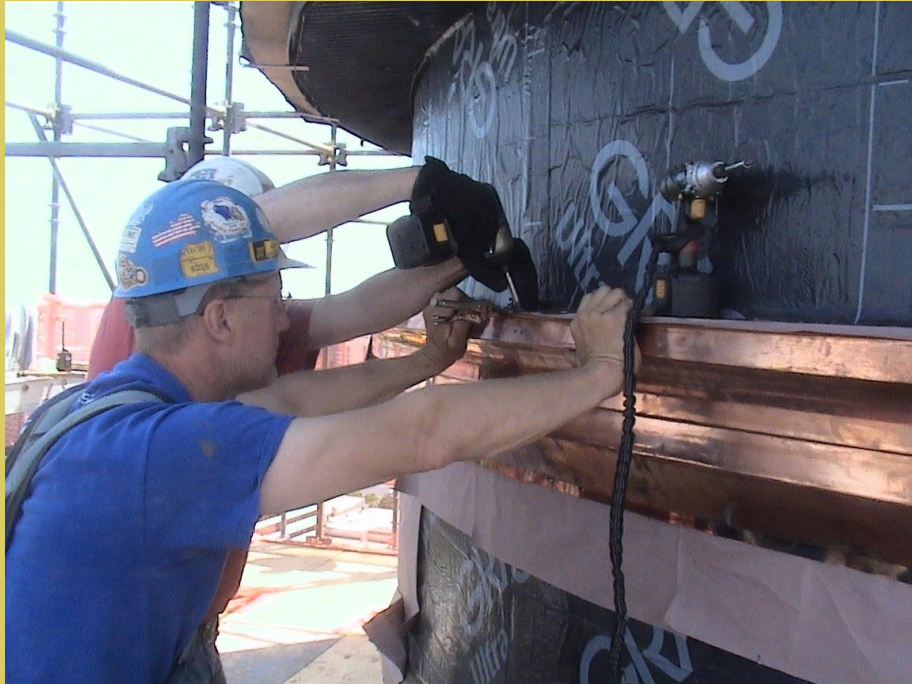
Installation of copper course on south tower drum.
