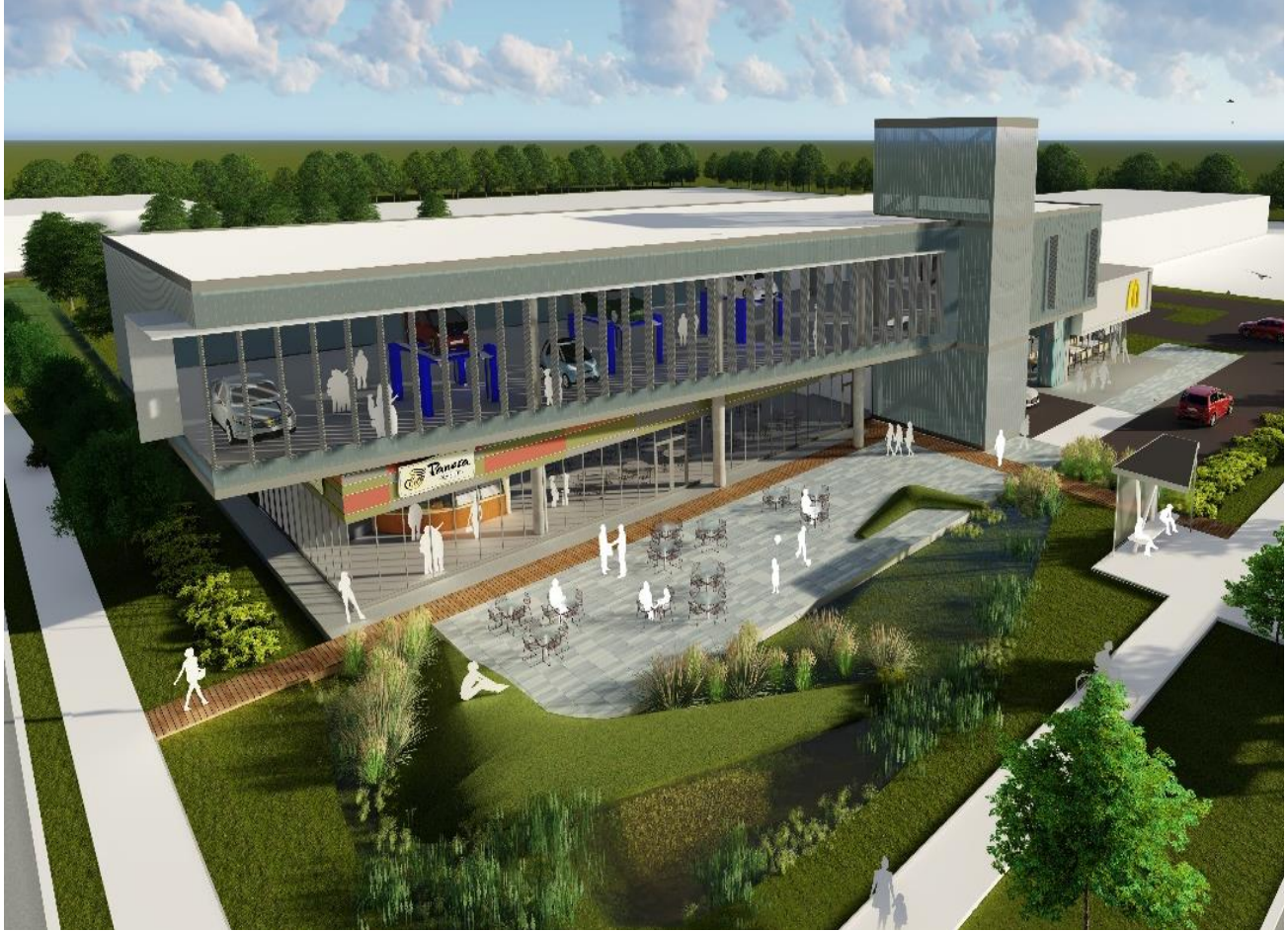
Eppstein Uhen's design engages a critical intersection along South 27th Street, providing new retail and office space while retaining the existing McDonald's (Credit: UWM Community Design Solutions and Eppstein Uhen Architects)
