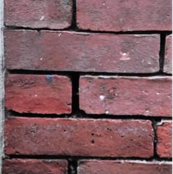
Brick foundation to be tuck pointed and repaired
