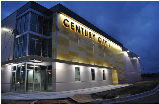
Construction draws to a close at the Century City I building, part of the Century City Business Park, which will attract new industry to Milwaukee's near north side. (Source: Redevelopment Authority, City of Milwaukee)
