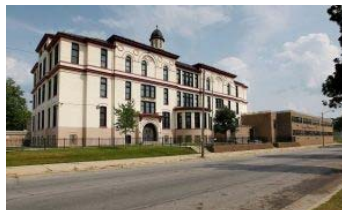
The former Phillis Wheatley Elementary School, 2442 N. 20th St., is being converted into affordable apartments with help from the city. A new report says Milwaukee's affordable-housing programs need more efficiency and private-sector money. (Photo courtesy of the Milwaukee Journal Sentinel)
