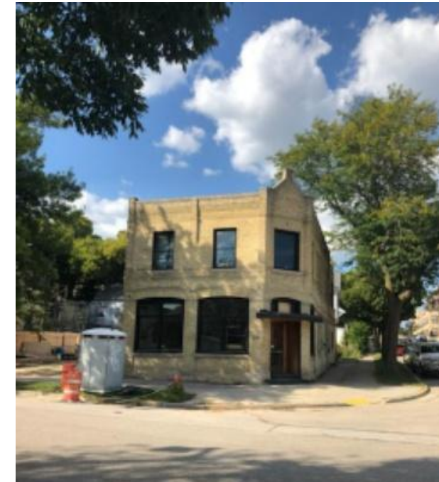
Facing North / South face
