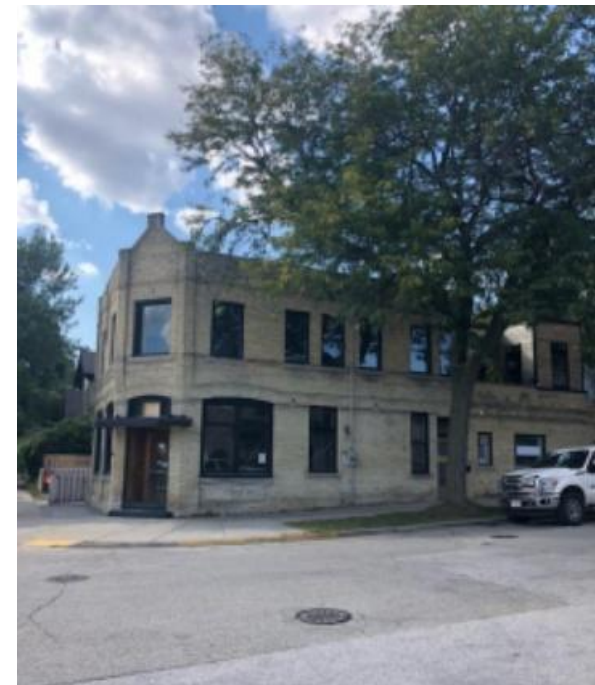
Facing west / East face
