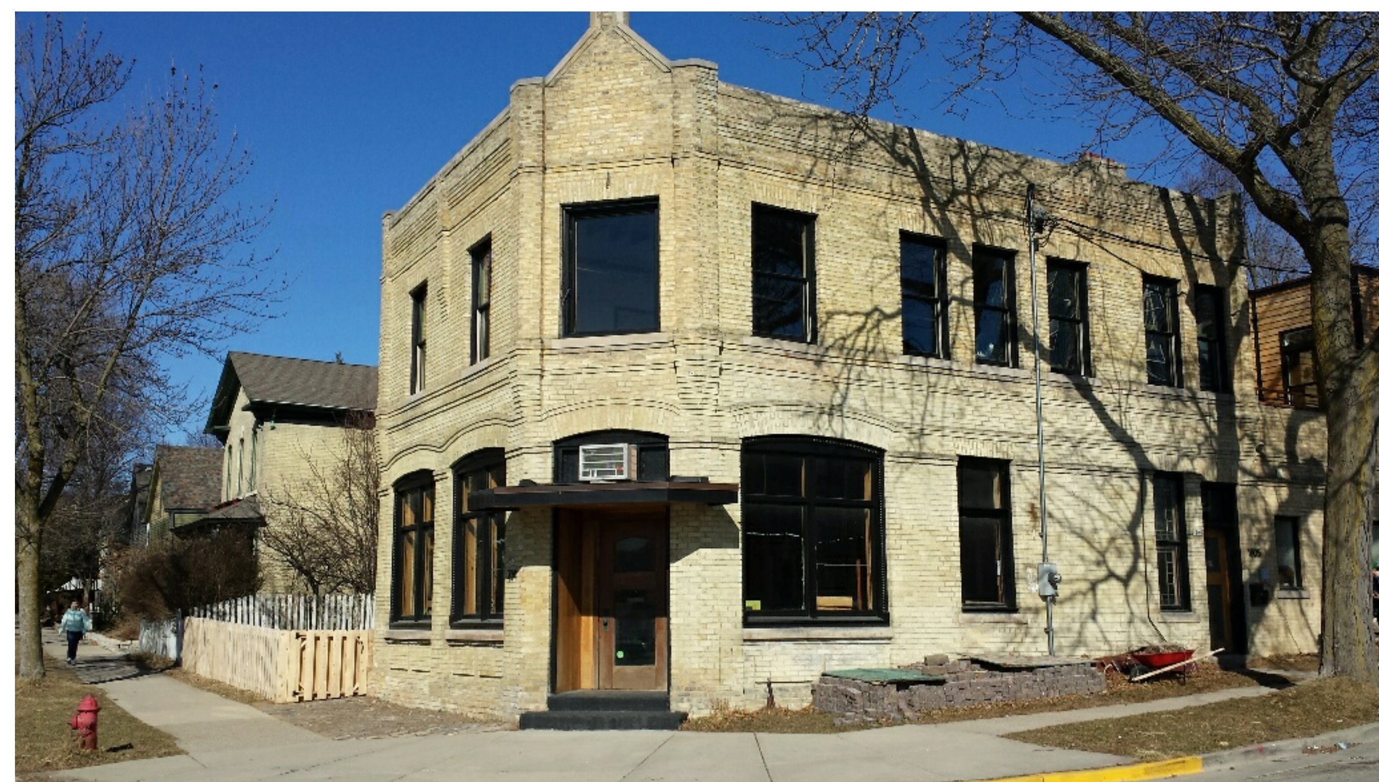
21 SE CORNER OF EXISTING BUILDING (FOR REFERENCE ONLY - NO WORK THIS AREA) 1/2" = 1'-0"
