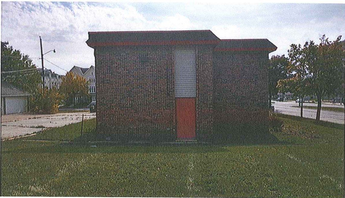
North façade of existing building looking south
