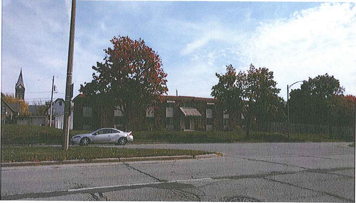
Looking east from 6 th Street
