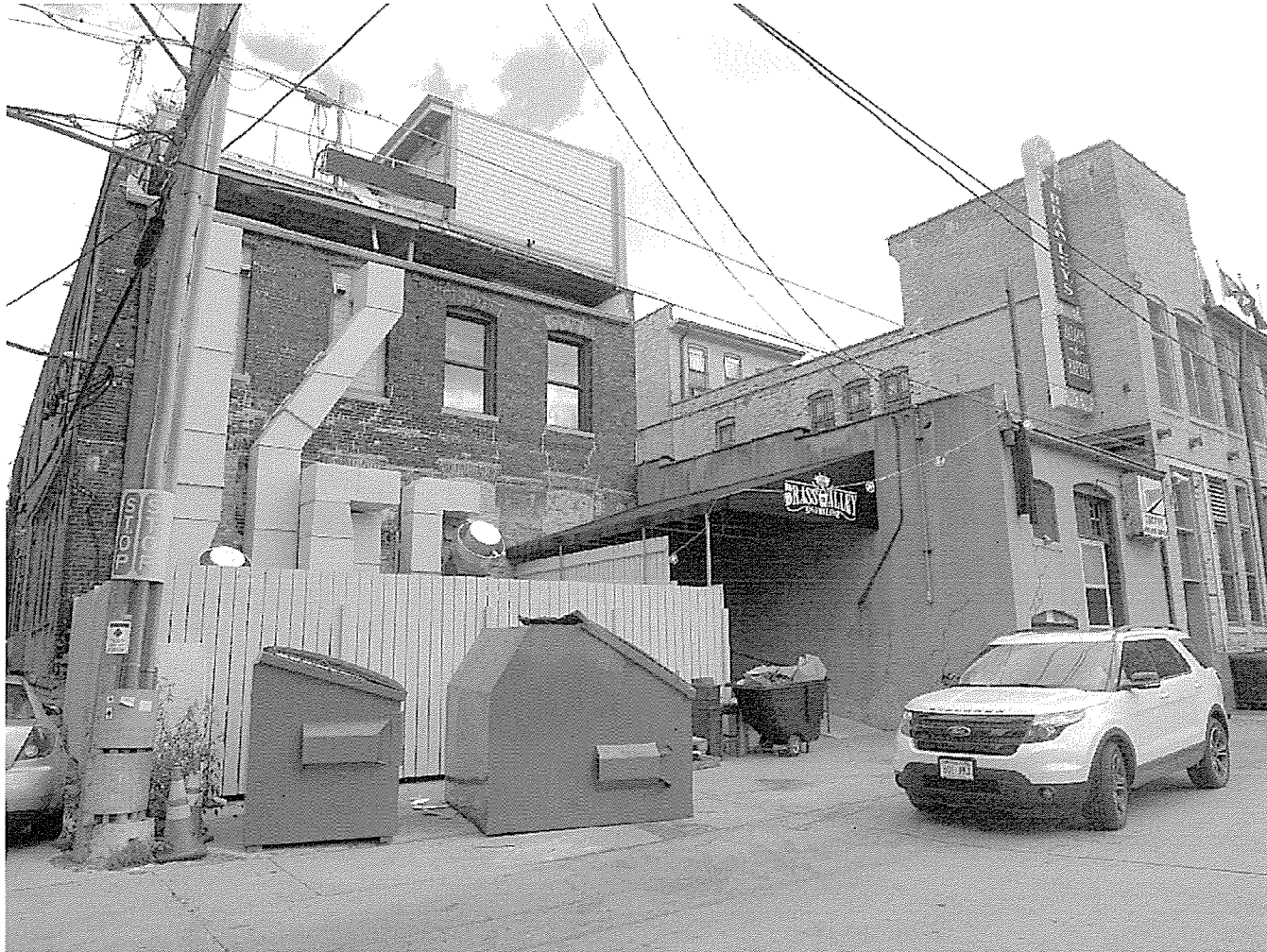
West elevation looking east
