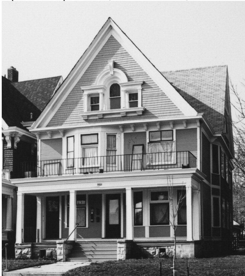
House in 1984 with no ground floor railing.
