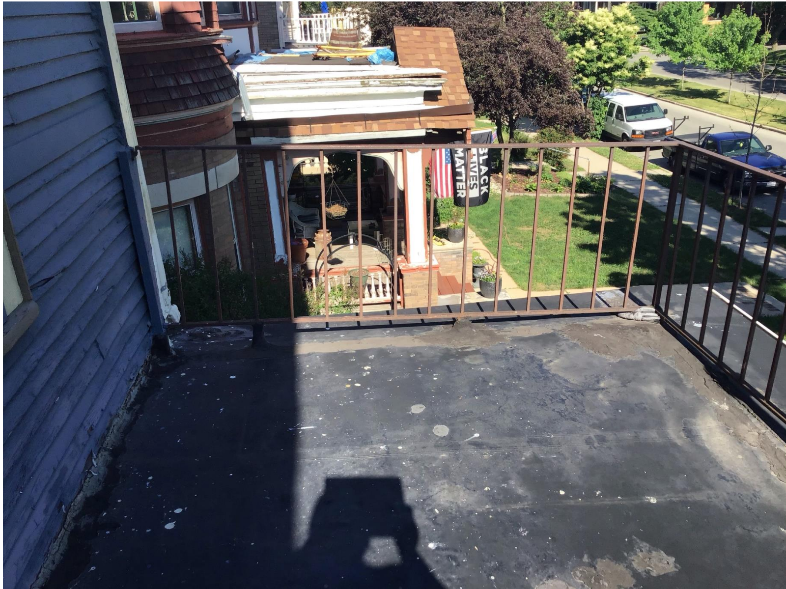
Typical balcony condition
