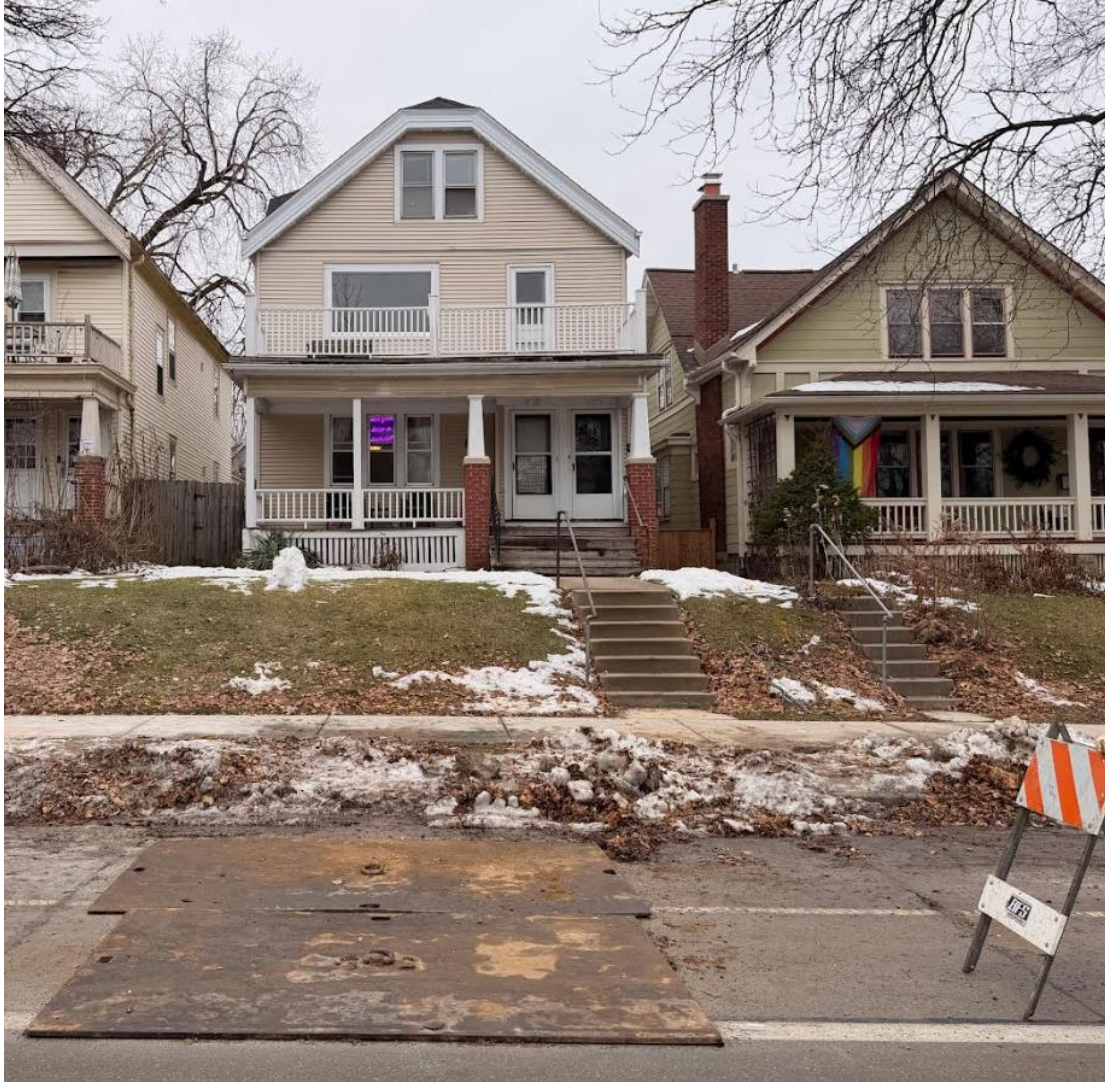
Photo showing excavation location at 3149/3151 N. Humboldt
