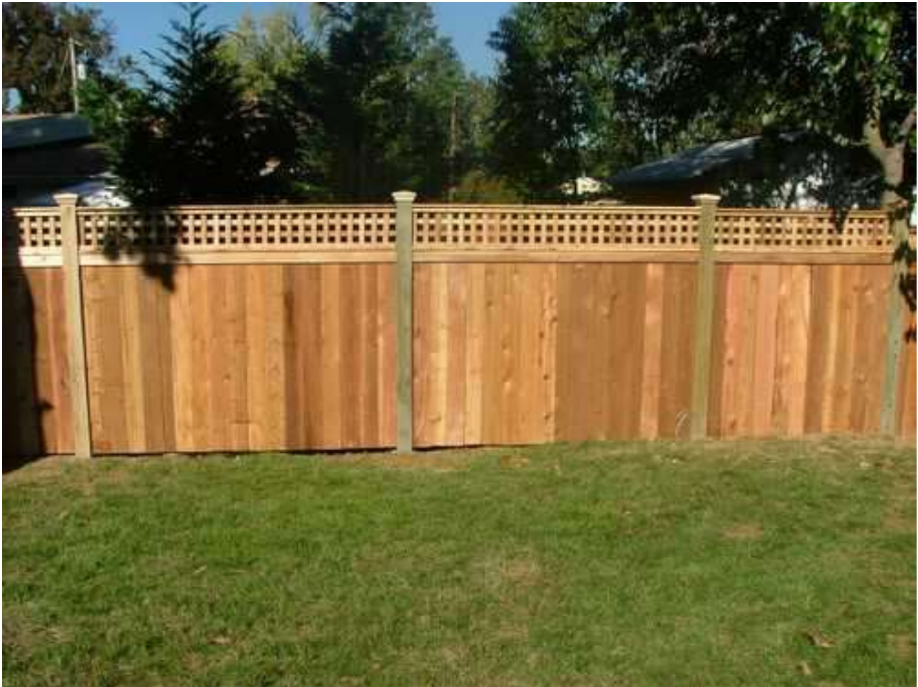
Fence for property line, must be painted or treated with an opaque stain.
