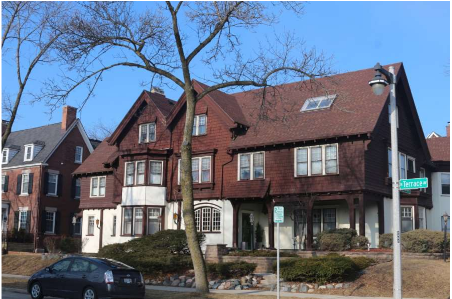
Terrace Avenue View showing skylight to be replaced with dormer.
