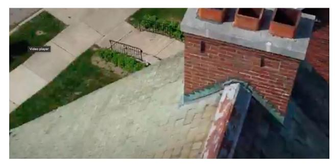
This photo shows properly placed step-flashing in copper. This technique must be copied with any replacement flashing anywhere on the building. Other forms of flashing into masonry are not acceptable.
