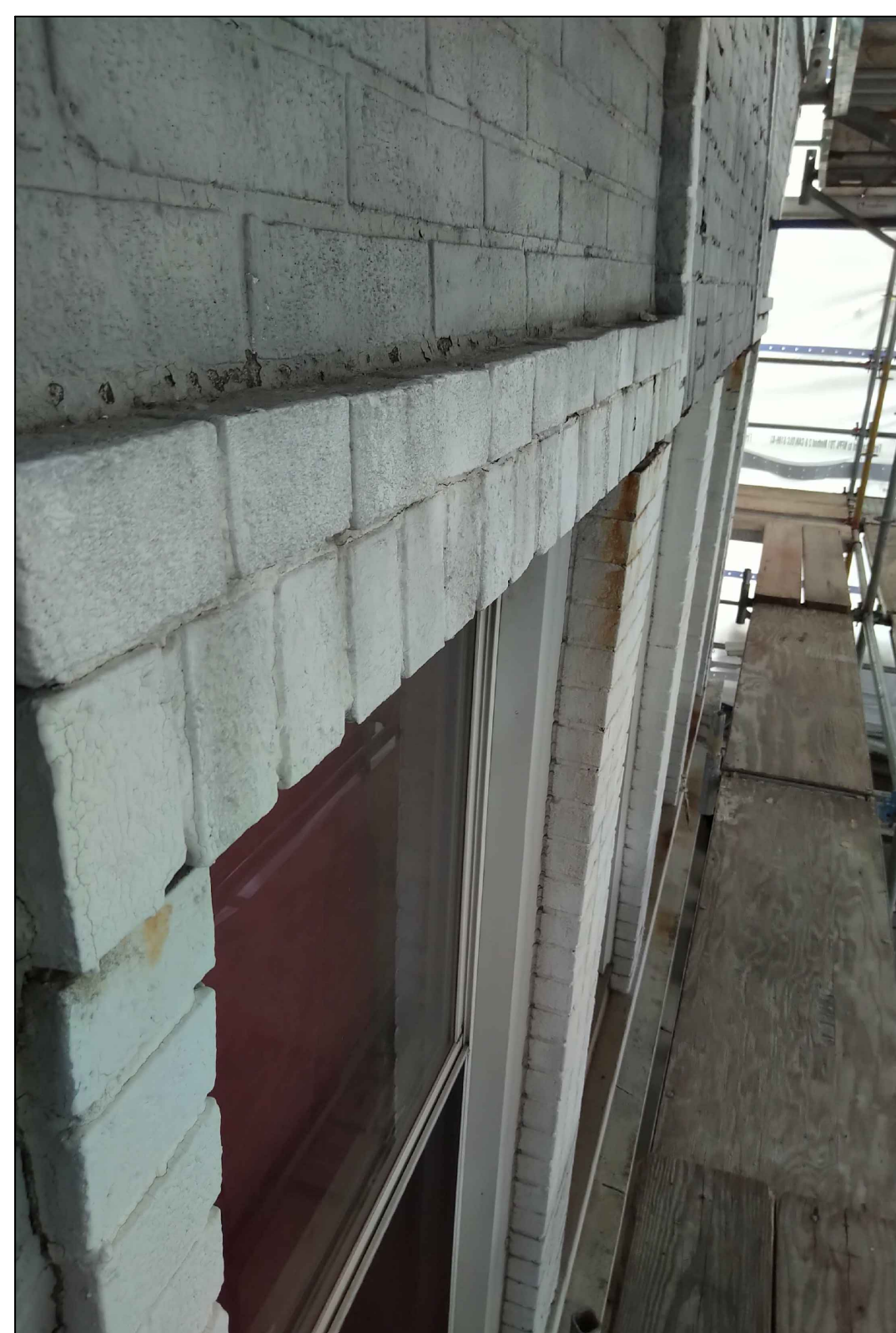
UPPER WINDOW HEADER BRICK DETAIL
