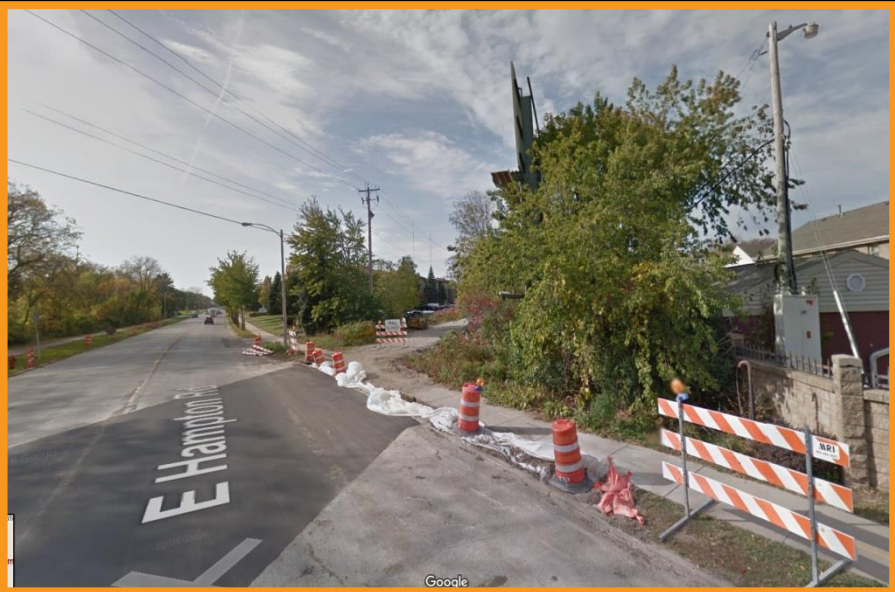
View from E. Hampton Ave. facing northwest
