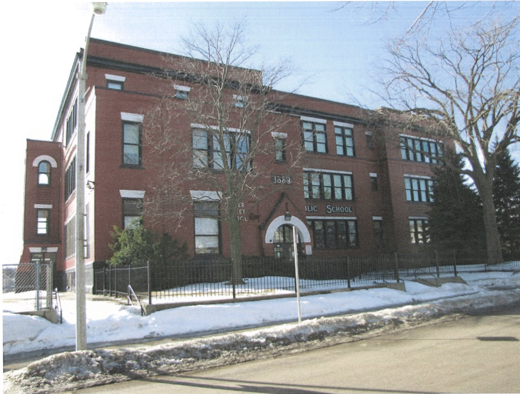
E. DOVER STREET AT DOVER STREET SCHOOL ENTRANCE.
