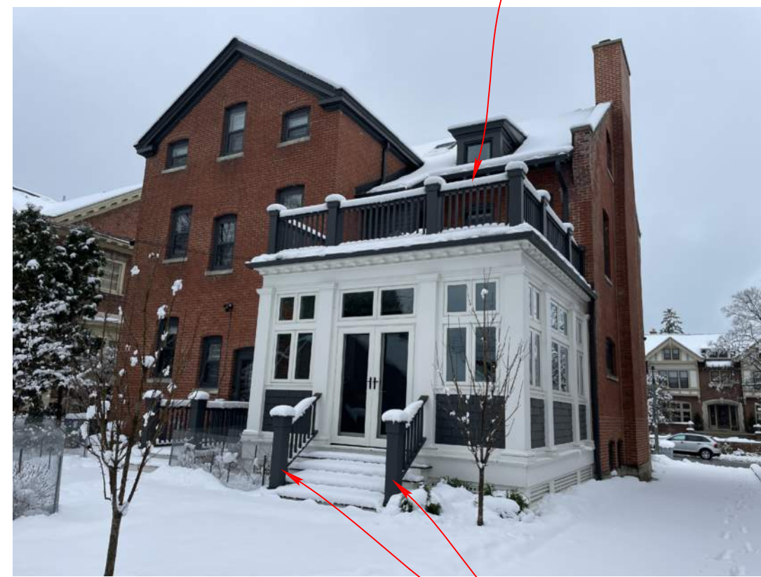
PHOTO 3 REAR PORCH AS SEEN FROM BACK YARD
