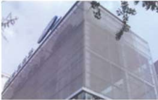
BACKLIT PERFORATED METAL PANELS WRAPPING FINGERS AT PRECAST BASE AND ILLUMINATING LANDSCAPING BELOW
