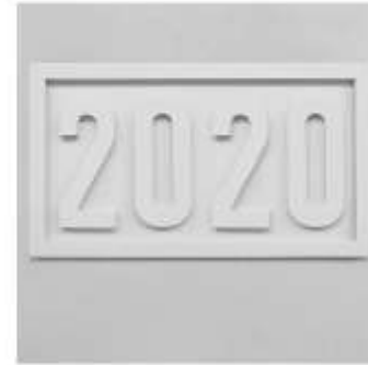
BUILDING NAME / ADDRESS CAST INTO CIP CONCRETE WALL PANEL
