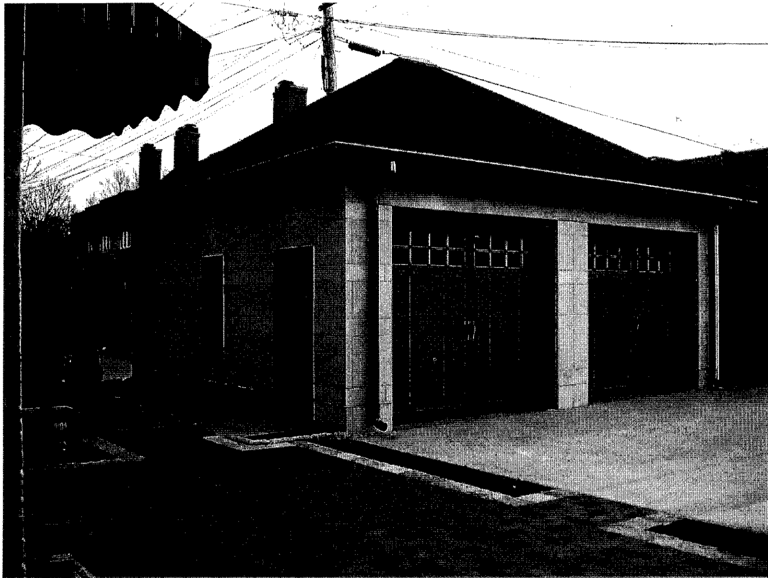
New Garage with Bedford Limestone cladding
