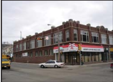
Renovated apartment units over commercial space on North Ave., with new townhouses along 35th St.
